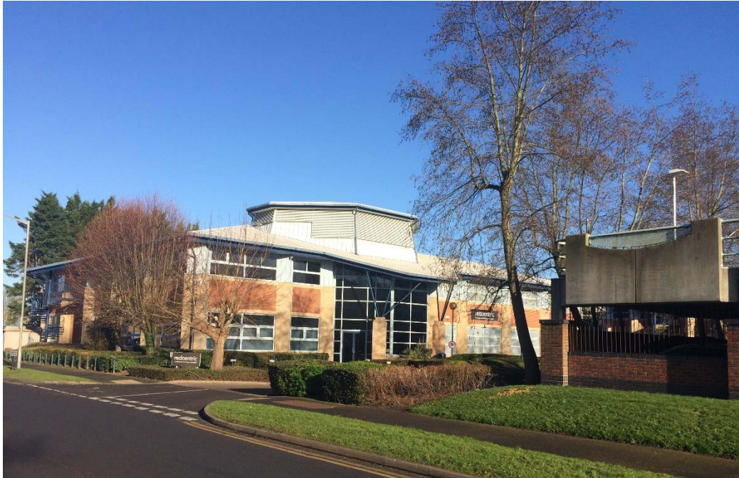
Image 4. View of the location for the gatehouse off Worton Drive
