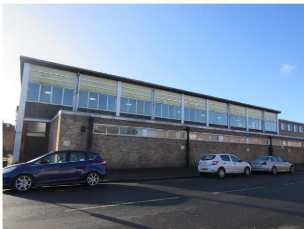
Photograph 3. Sections 1 & 2 of the building viewed from the north.
