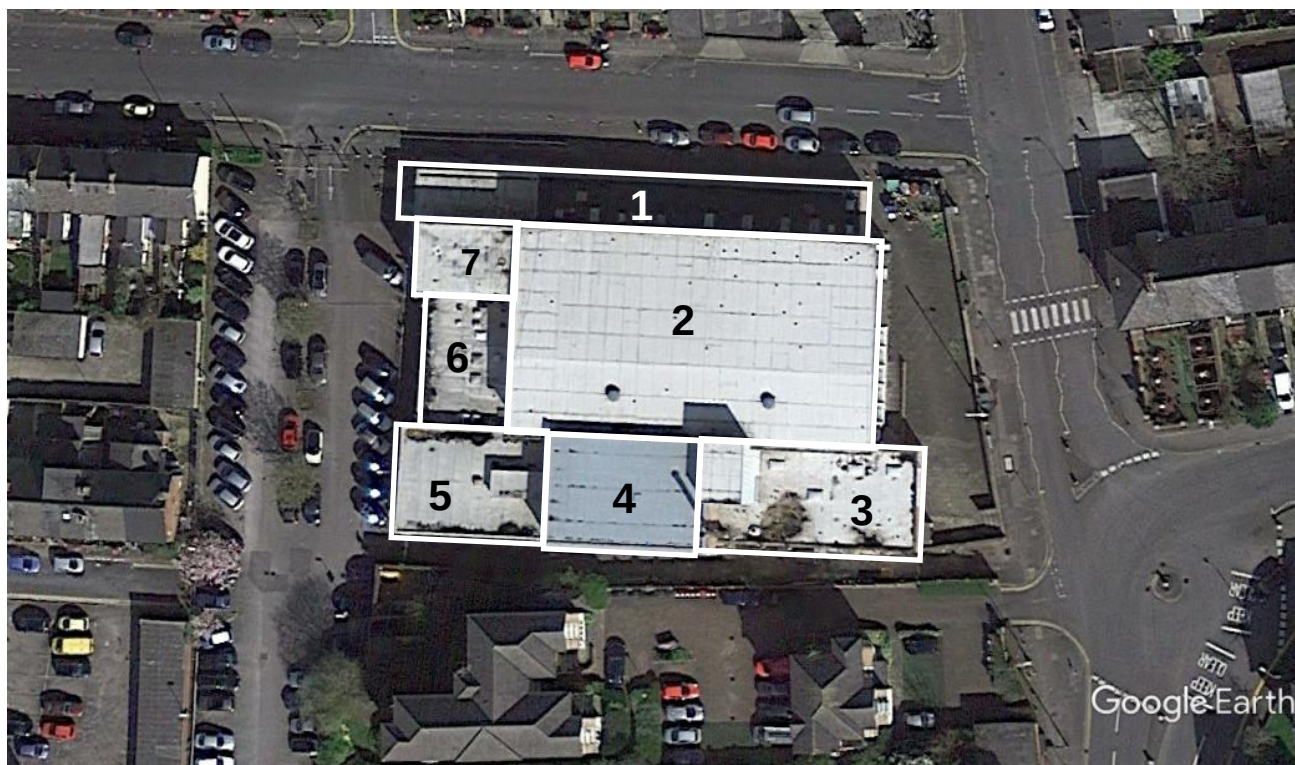
Figure 1. An aerial photograph of the building at the Central Swimming Pool, Reading. The different sections of the building are indicated and numbered; Section 1 to Section 7.
