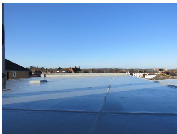
Photograph 8. The roof of Section 4 of the building (looking west).
