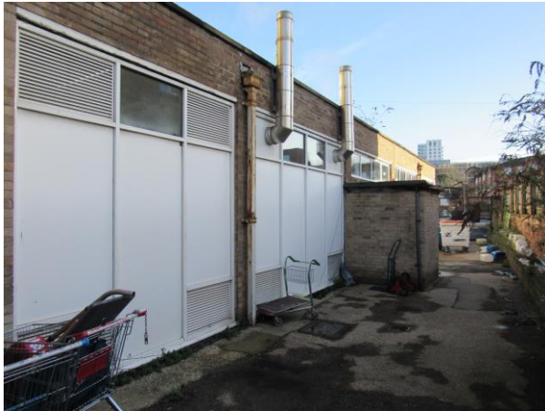
Photograph 9. The southern elevation of Section 3 viewed from the south.
