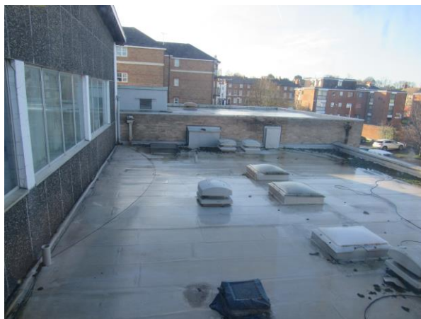
Photograph 2. The flat roof of Section 6.
