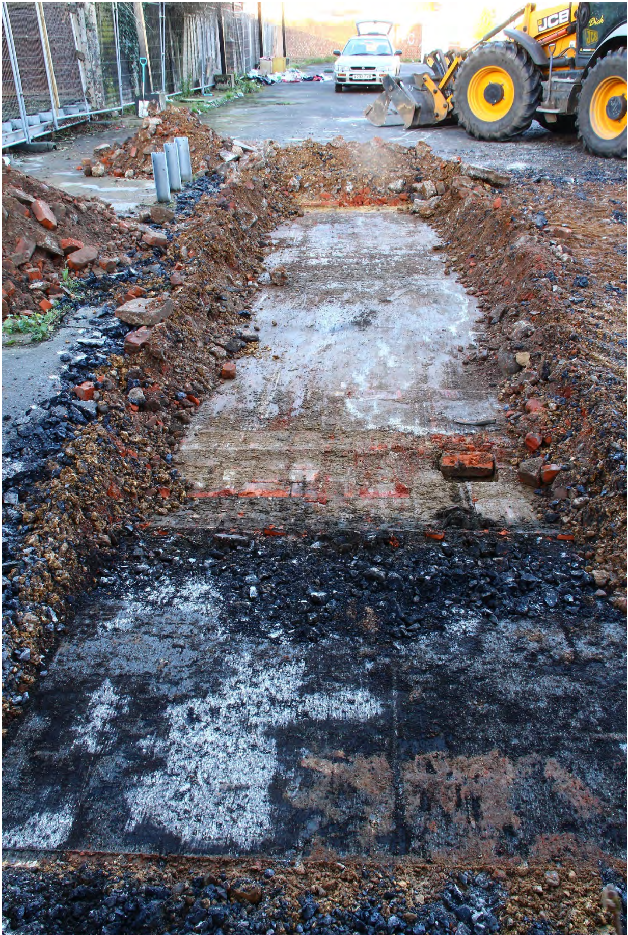
Above, the remnant foundation and floor slab of the former building on the site
