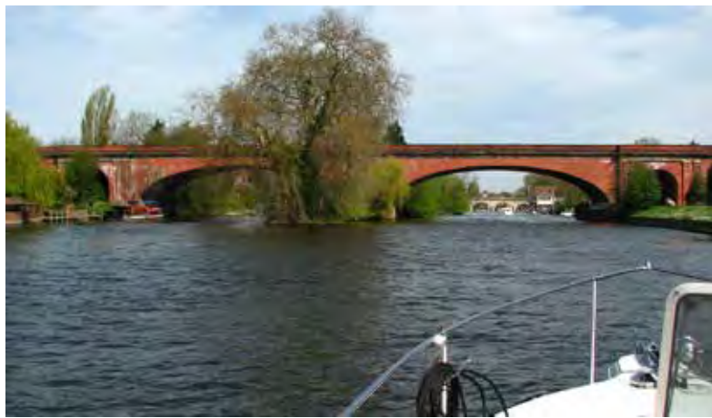
Figure 49. Maidenhead Railway Bridge
