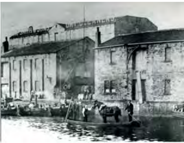
Figure 48. Horse Ferry at Reavensthorpe (Yorkshire Waterways Museum).
