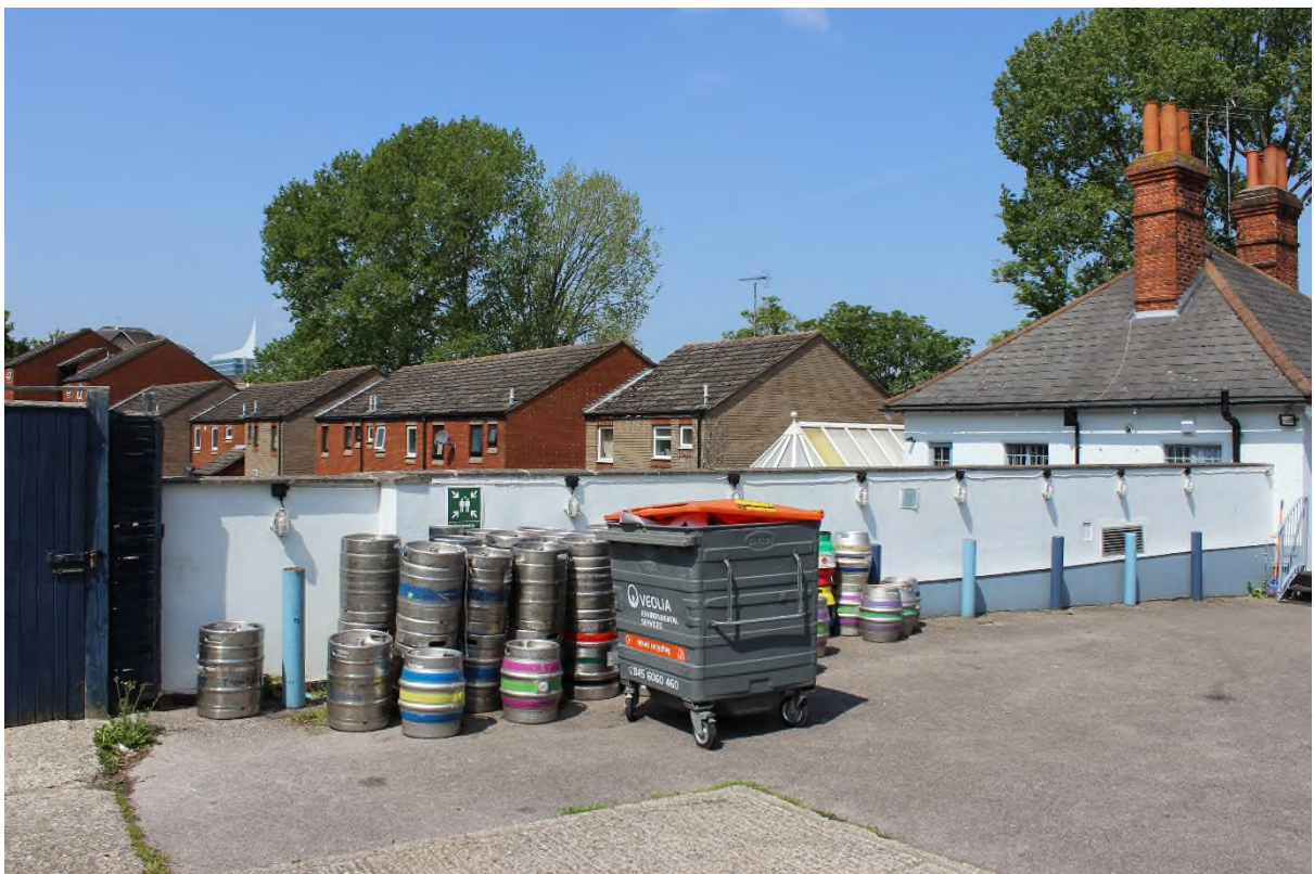
Figure 5 View to the rear elevation from the car park. The boundary wall is the upper part of the rear wall of the cellar range.
