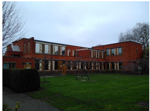
Building LO33, looking North-East
