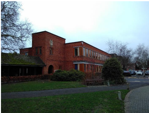
Building LO33, looking South-West
