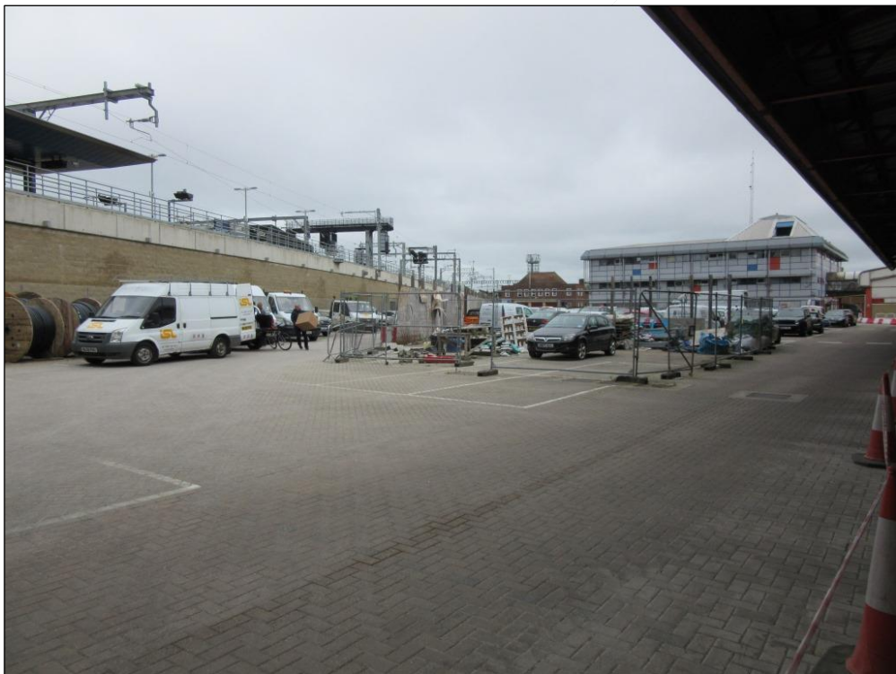
Photo 1 General view of the Site
