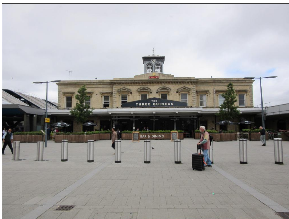
Photo 2 Main Building at Reading General Station as seen from the pedestrian area to the south
