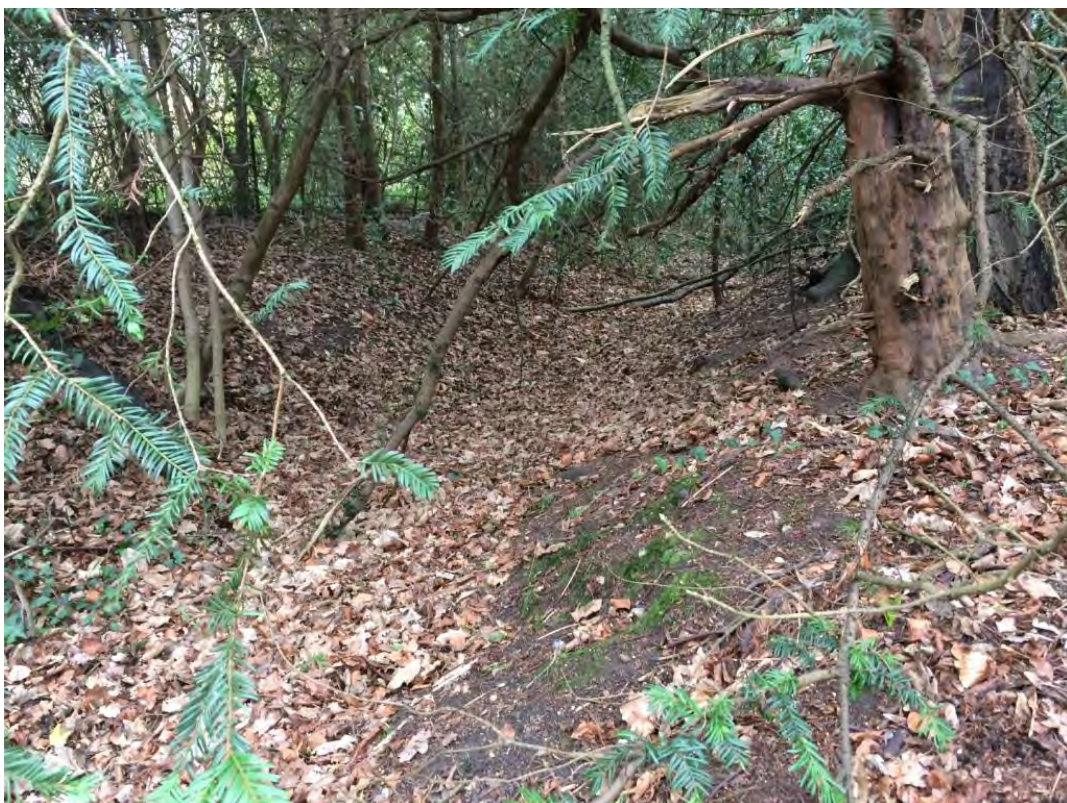
Photo 13 – Start of drainage ditch approx. 175m south-east of the site. Observed as dry and does not appear to have received water for some time.
