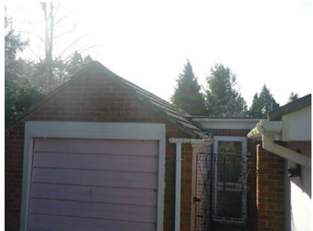
Photo 4: Northern elevation of Garage
