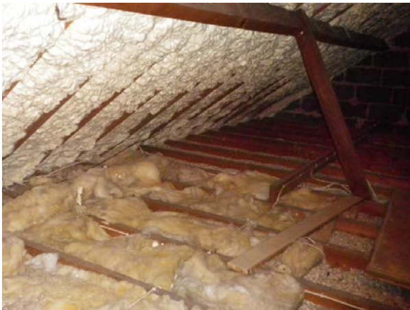
Photo 3: Interior of Bungalow roof space
