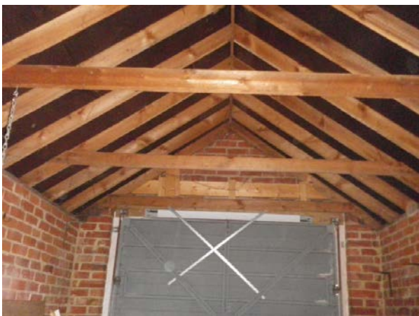
Photo 5: Interior of Garage
