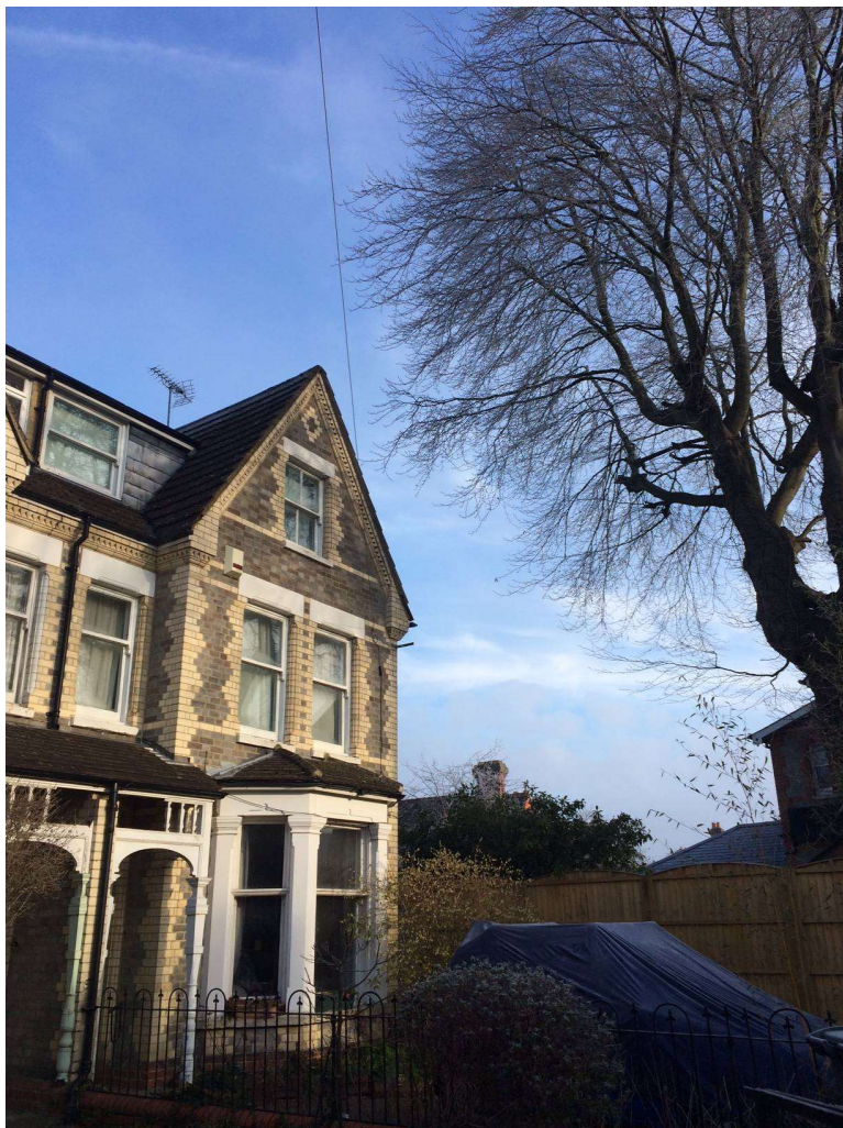
Proximity to 90 from Crescent Road
