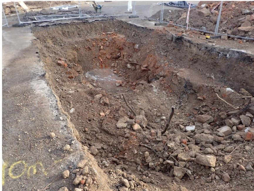
Plate 4: View E, demolition material over concrete floor Trench 3
