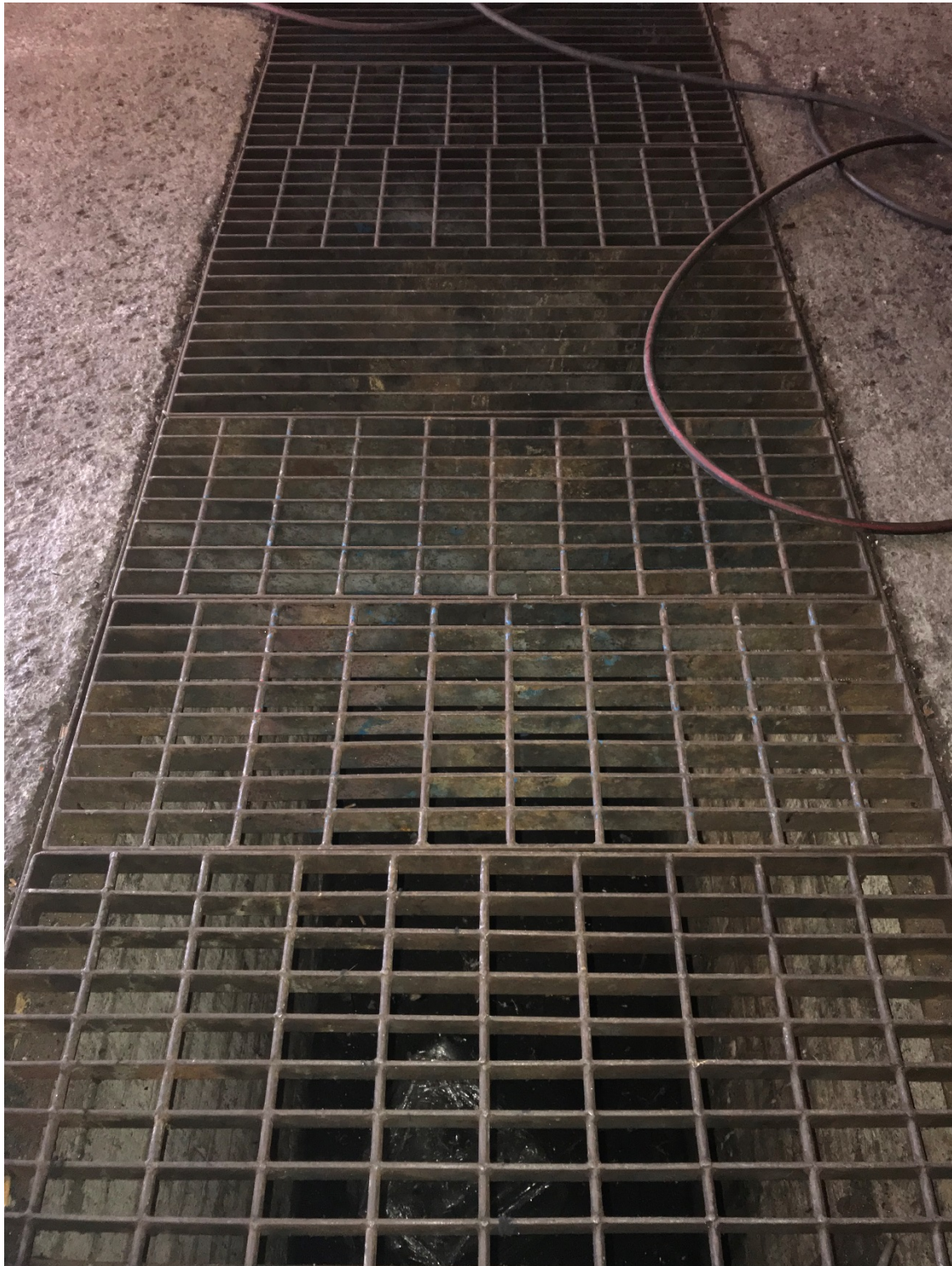
Inspection pit within tyre fitters
