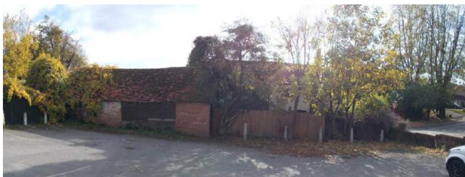
Plate 3: The southeast boundary of the Site, from the centre of the car park.
