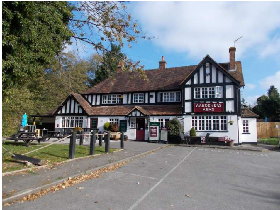
Plate 2: The front elevation of the Gardeners Arms.
