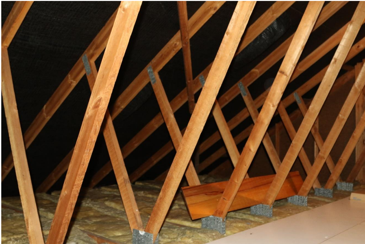
Image 7 – Additional view from within the roof void demonstrating a felt membrane below the roof coverings, insulation to the floor coverings with timber boards across the central areas.
