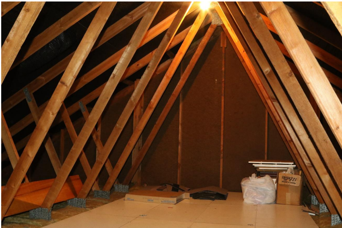
Image 6 – Internal view from within the roof void
