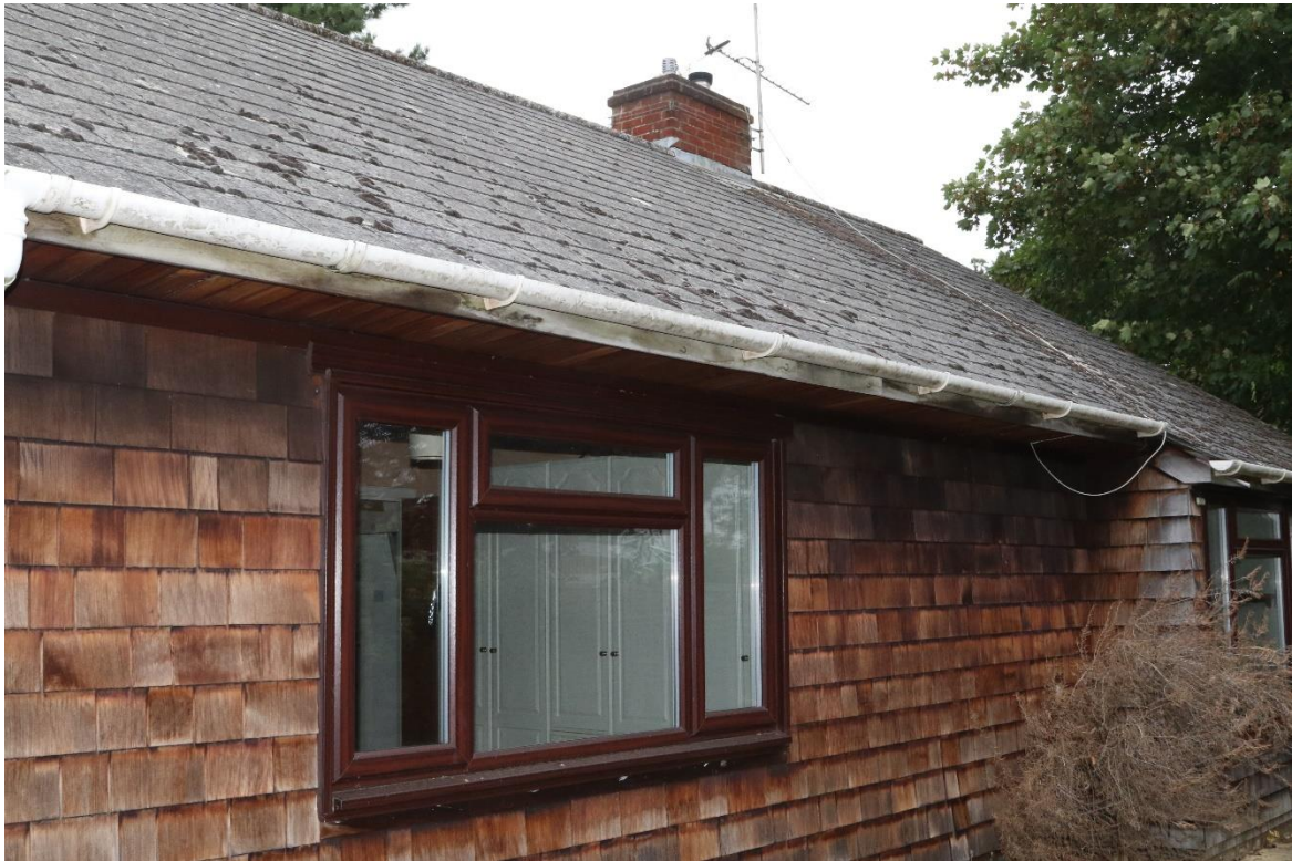
Image 5 – South facing elevation of the building
