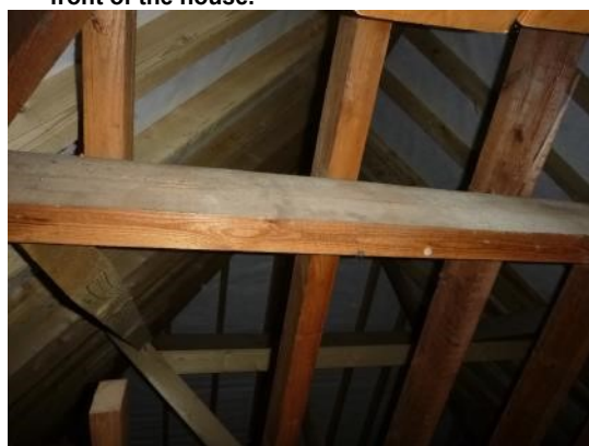
10. Internal view of the roof space showing the junction between more modern extension and original section of the roof.
