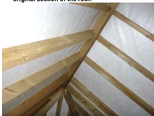
12. The northern end of the roof space lined with breathable membrane.
