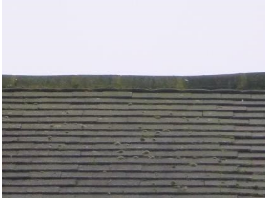
3. Row of curved roof tiles visible just below the ridge at the front of the house.
