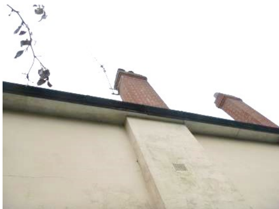
9. Soffit boxes tight around the eaves of the house.
