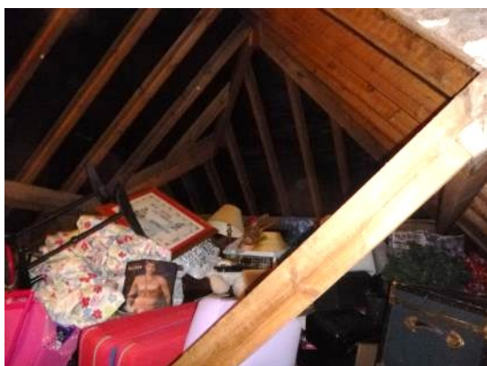
11. The main section of the roof lined with bitumen felt.
