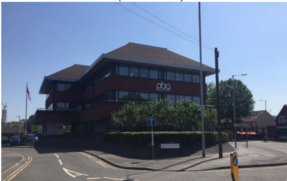
Photo 2 – Current Side Elevation (Caversham Road)
