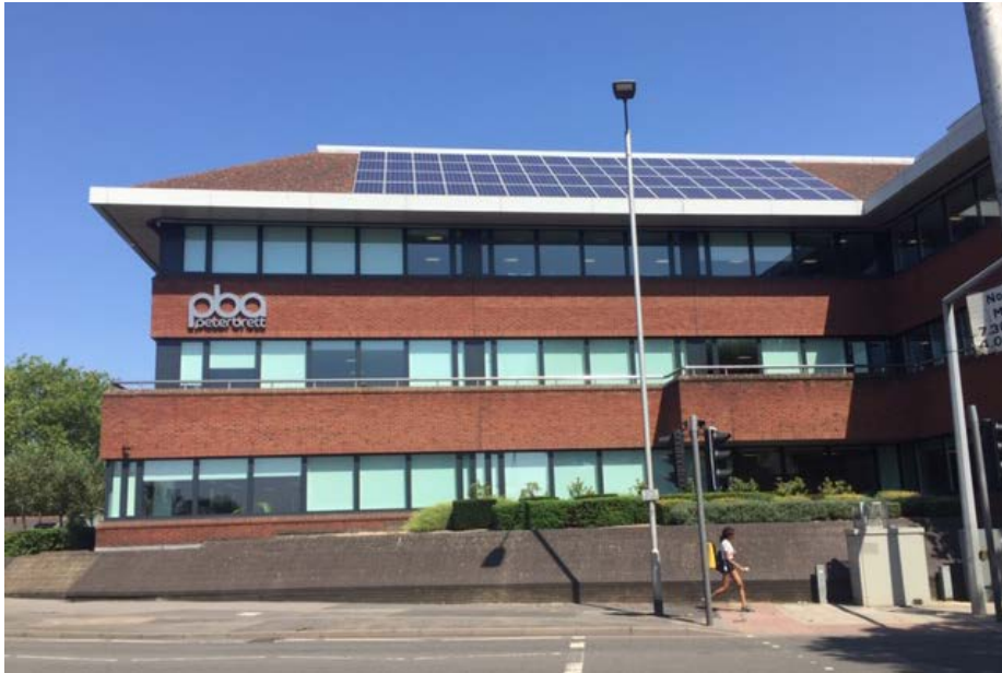
Photo 1 – Current Rear Elevation
