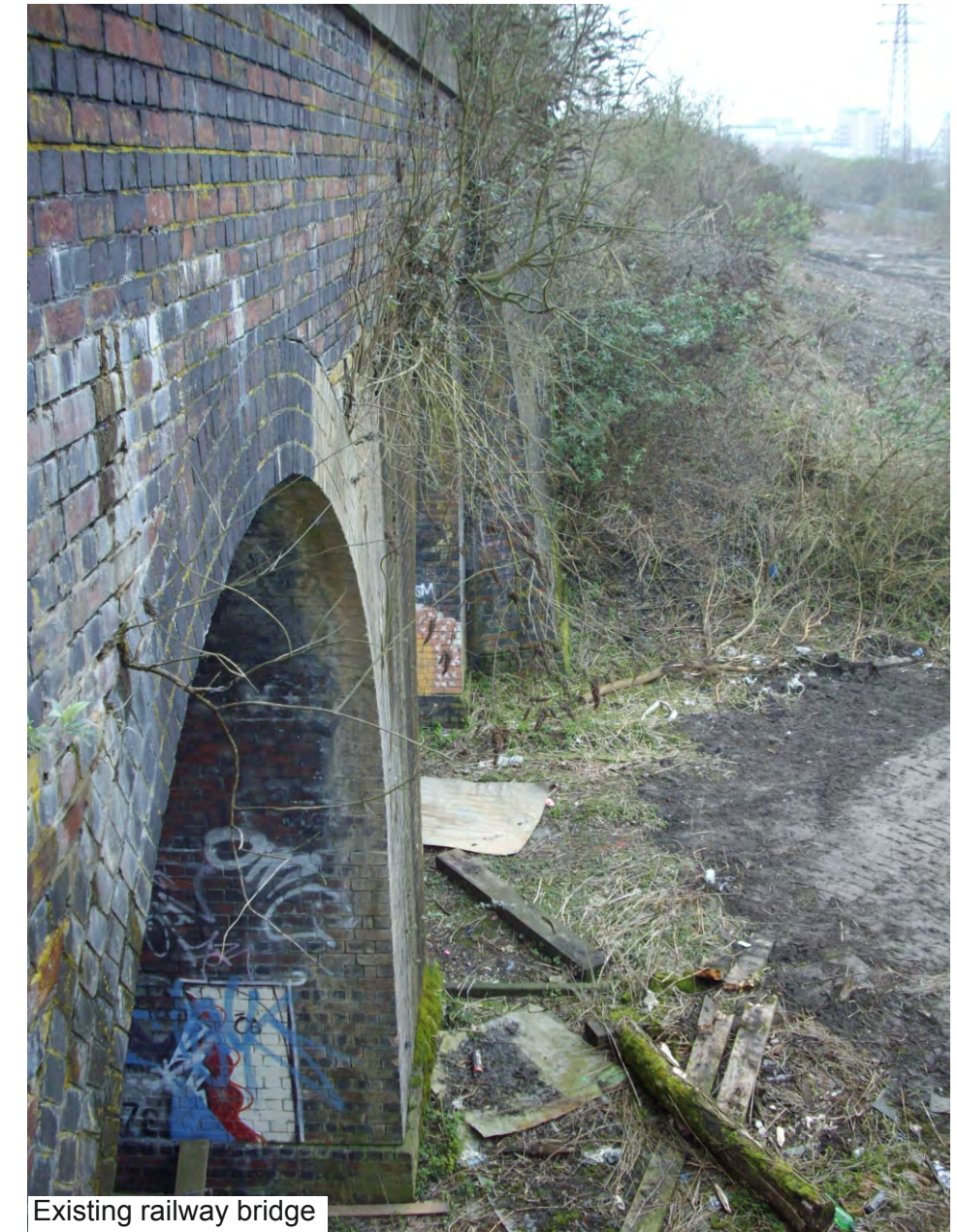
Existing railway bridge
