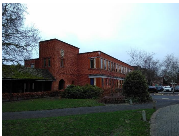
Building LO33, looking South-West
