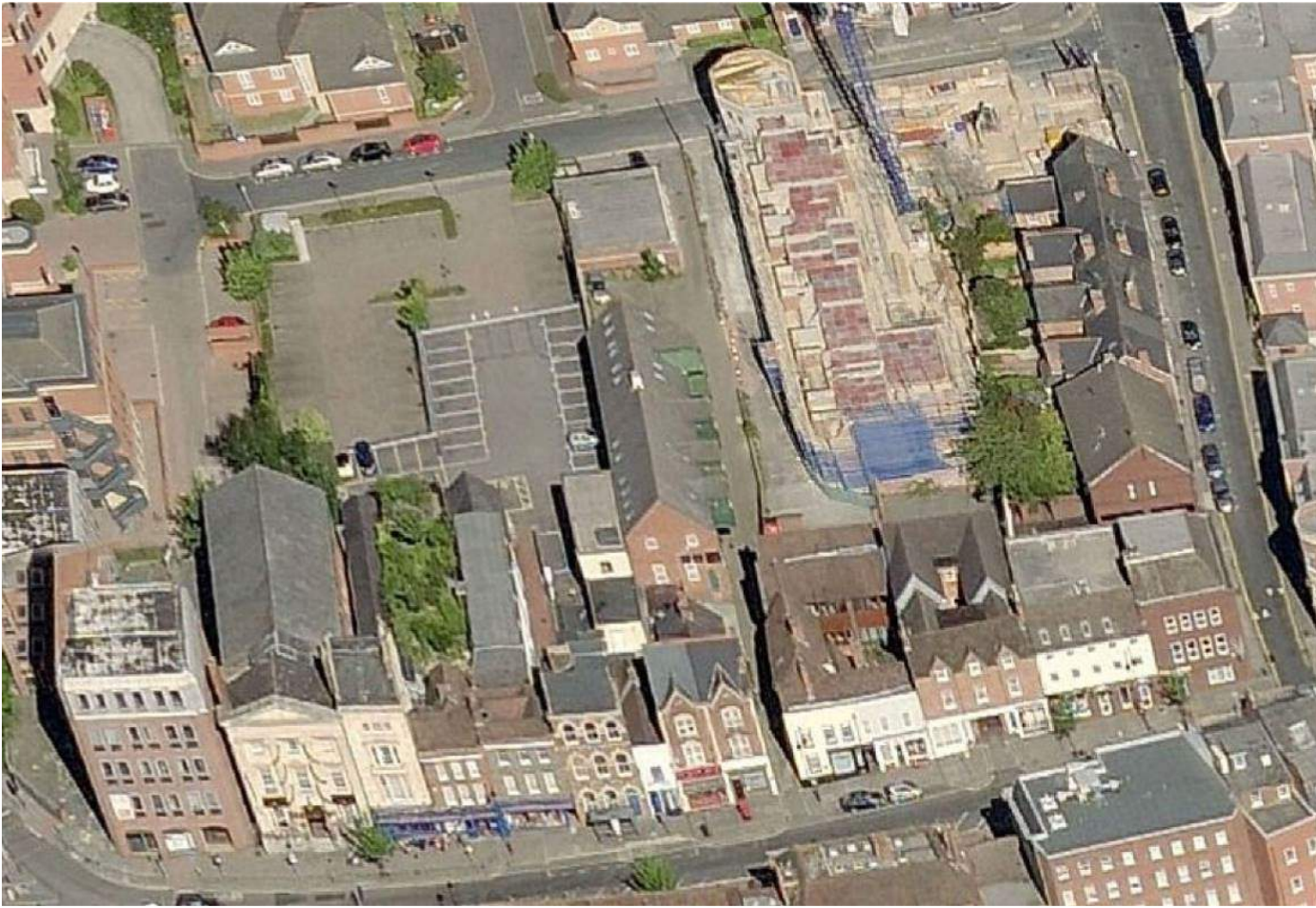
Figure 23 Aerial view – from west over London Street
