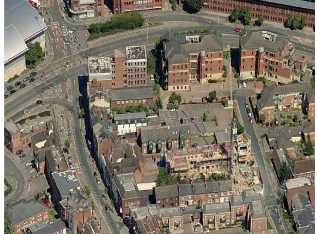
Figure 24 Aerial view – from south to Queen's Road
