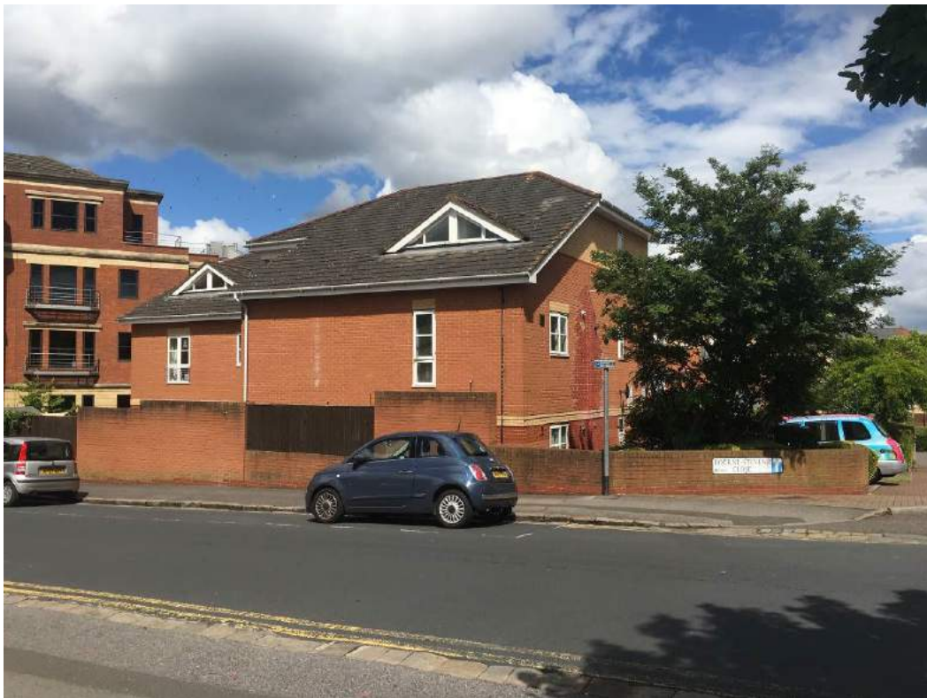
Figure 15 Gable of Bourne-Stevens Close facing site
