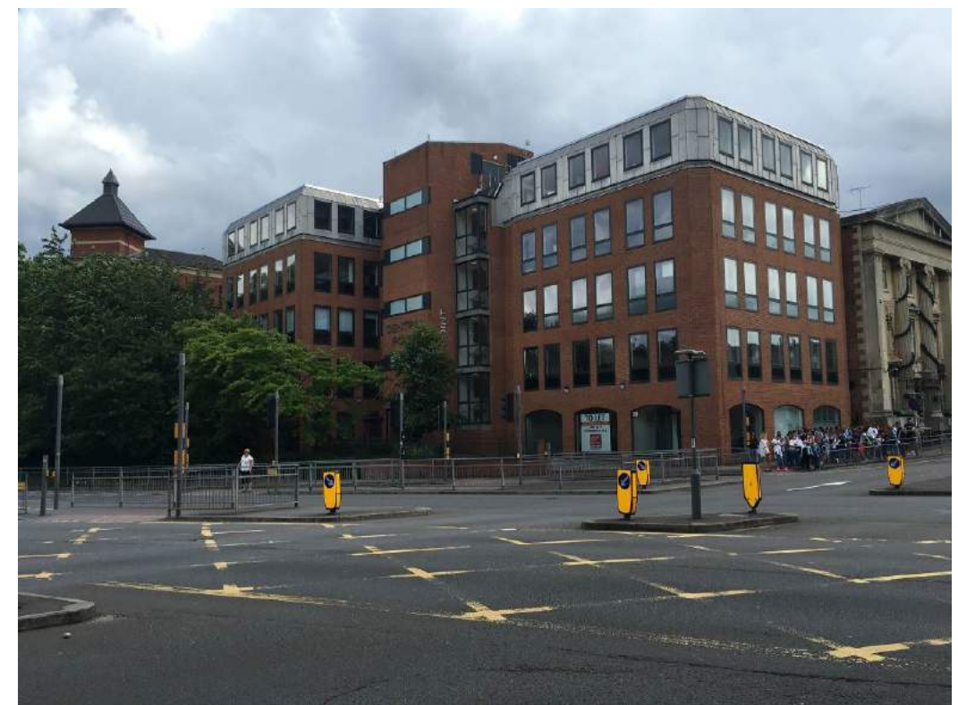
Figure 17 Offices at junction of Queen's Road and London Street
