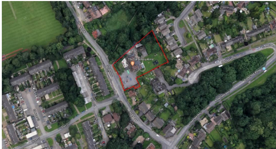
Figure 2: Site Location (Image courtesy of Google Maps)
