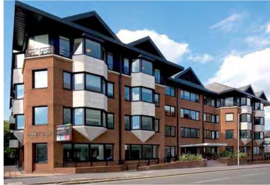
Figure 7. Existing Front Façade
