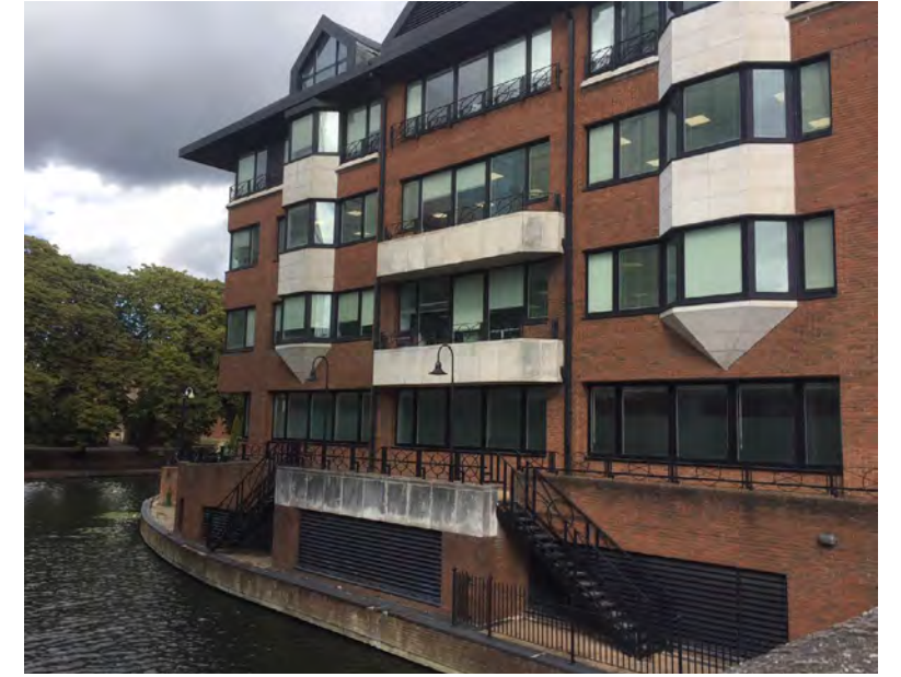
Figure 8. Existing West Façade
