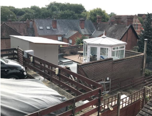
Existing roof-scape currently creating a negative impact on the surrounding area. Access to the existing house is via the cupola, roof terrace and shed further fill the space on the flat roof.
