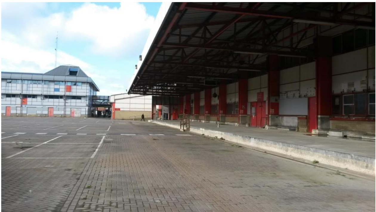
Photo 2: Raised concrete platform located to the south of the former sorting office.
