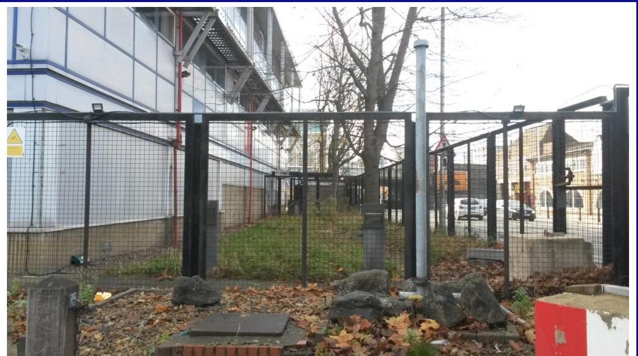
Photo 6: Ventilation pipe located behind three adjacent drains, indicating the presence of an oil/water interceptor.
