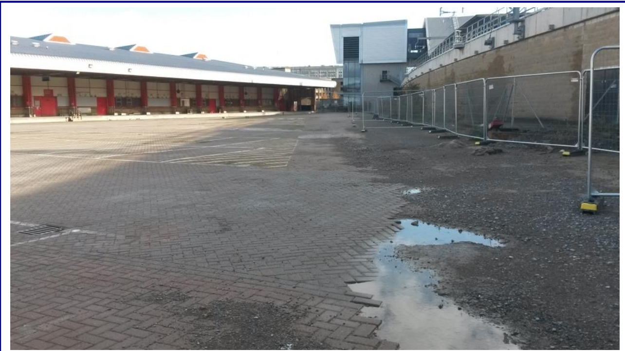
Photo 5: Southern boundary of the site with area of gravel.
