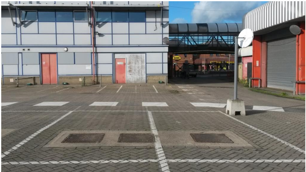
Photo 3: View of the office building to left with roller shutter doors of sorting office to right and walkway connected the two building in the background.
