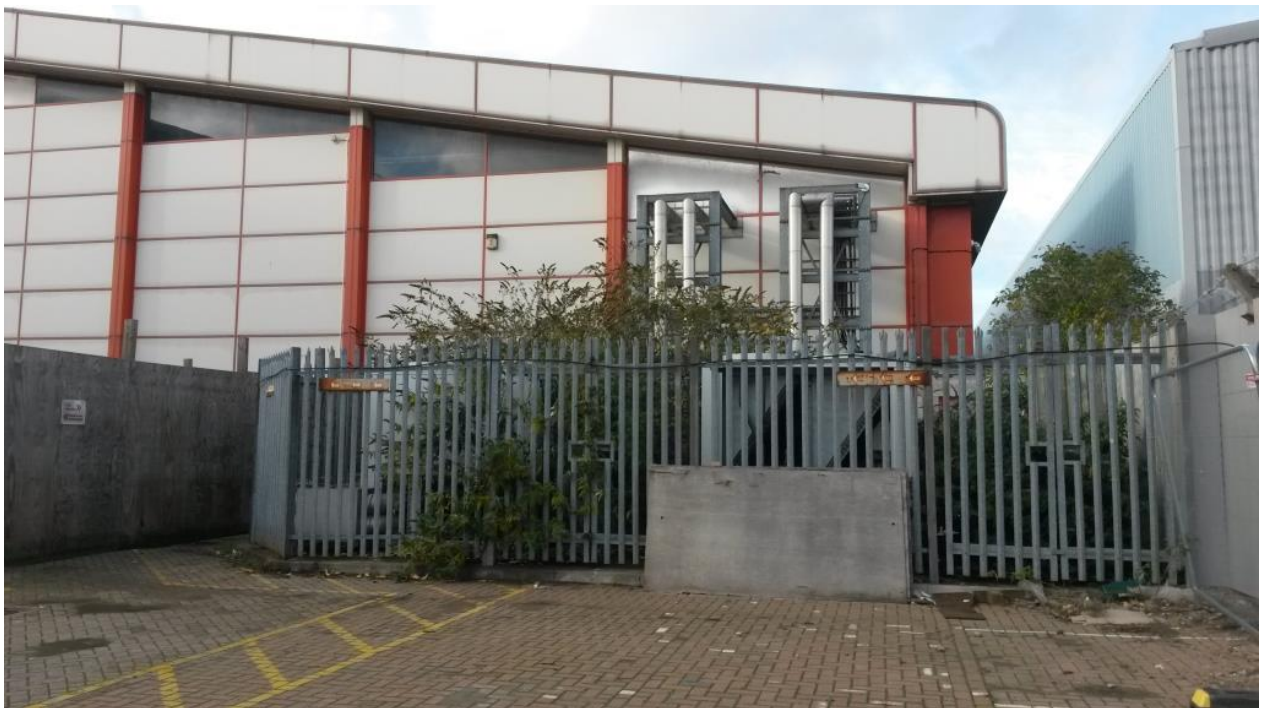
Photo 4: Overgrown likely former air handling equipment.
