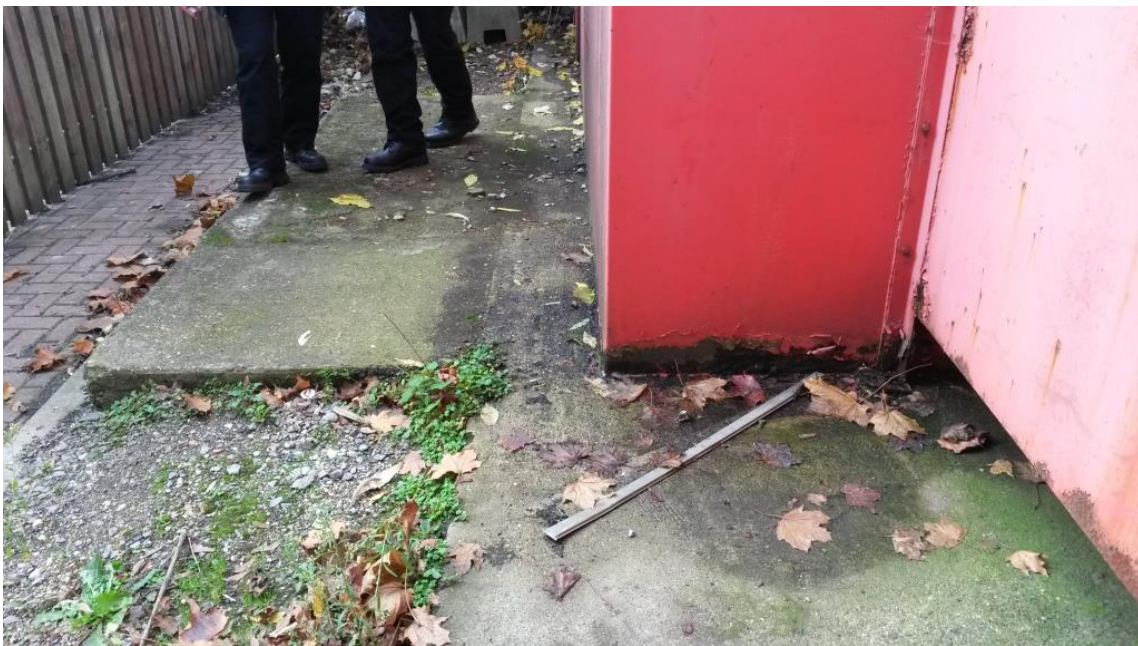
Photo 8: Minor staining noted on the concrete base externally to the generator unit.
