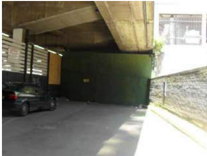
Entrance to Underground Car Park
