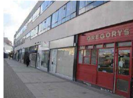
Station Hill Retail Units
