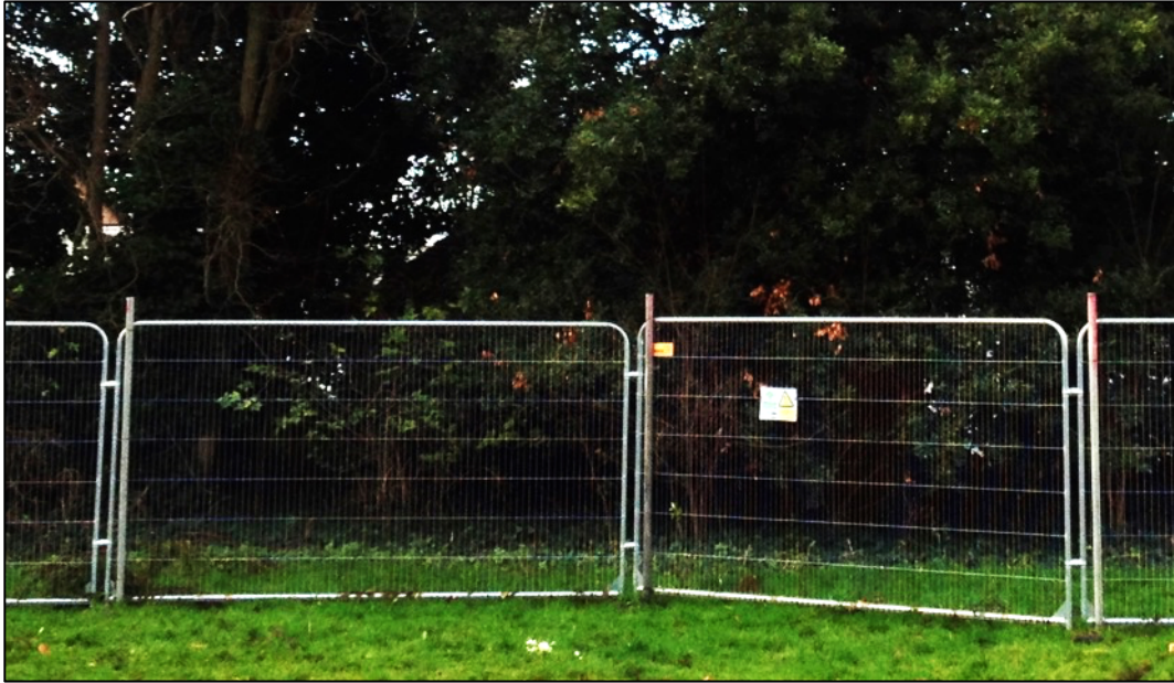
Weld-mesh panels on scaffold uprights
