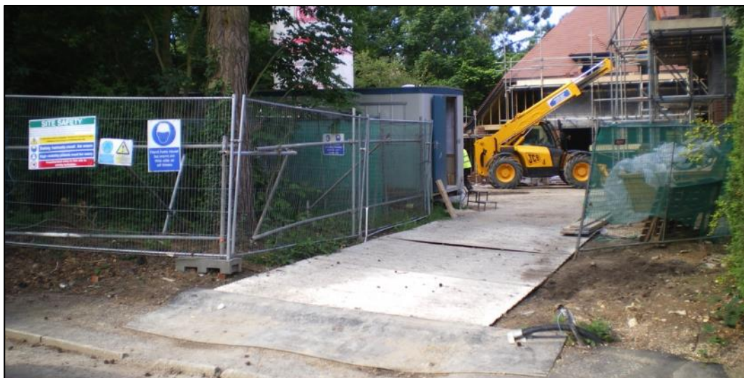
Vehicular ground protection trackway
