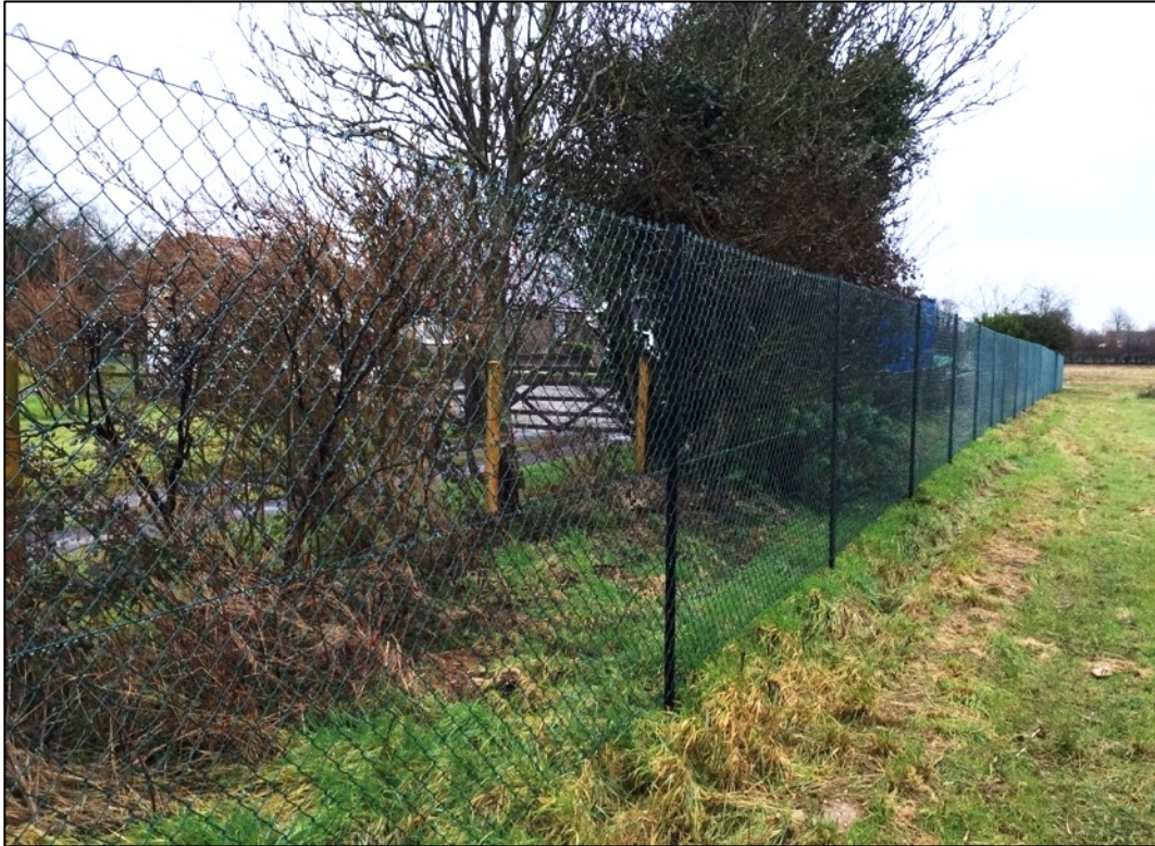
Chain-link on angle-iron uprights
