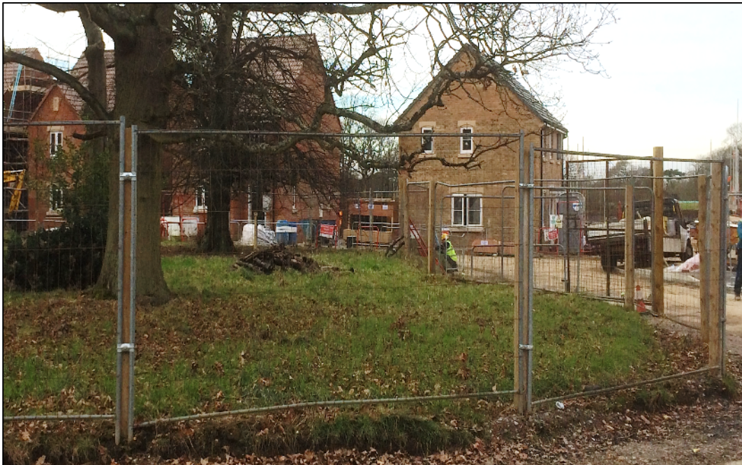
Weld-mesh panels on wooden posts
