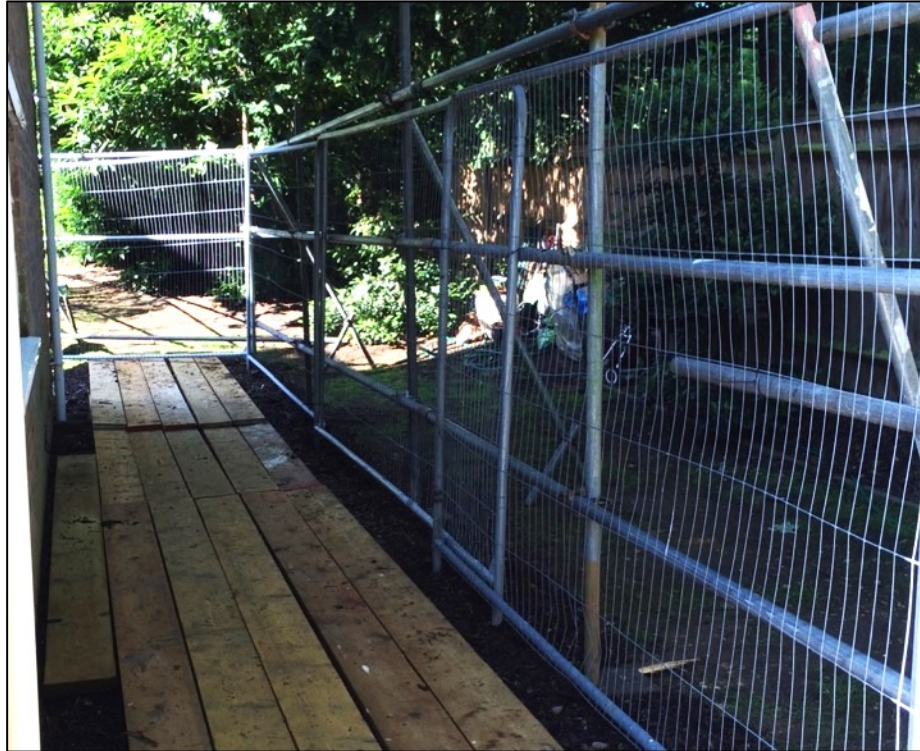
Scaffold board pedestrian ground protection
