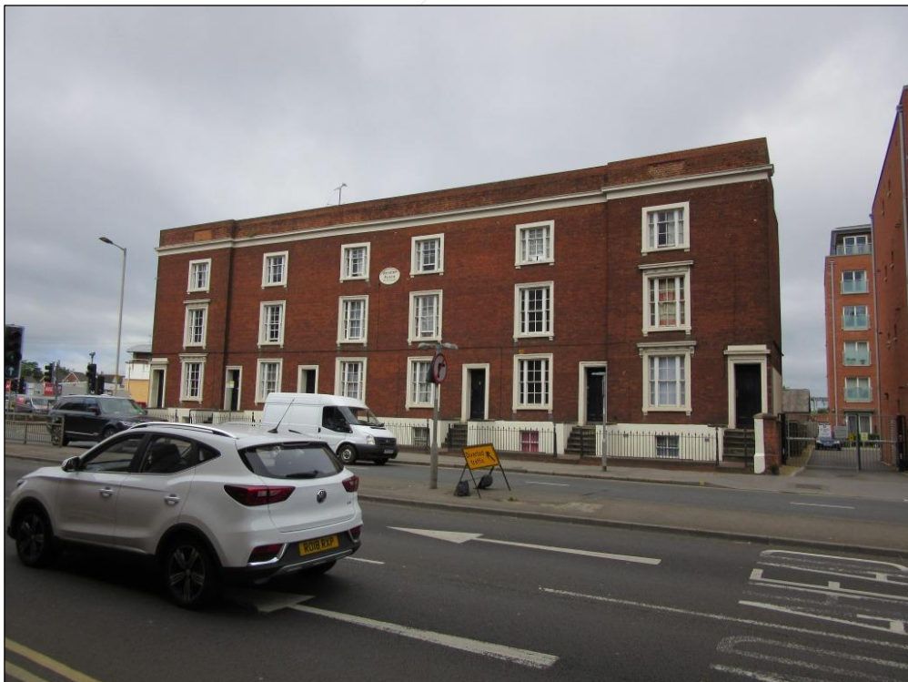
Photo 6 Regent Place as viewed from the north-east on Caversham Road
