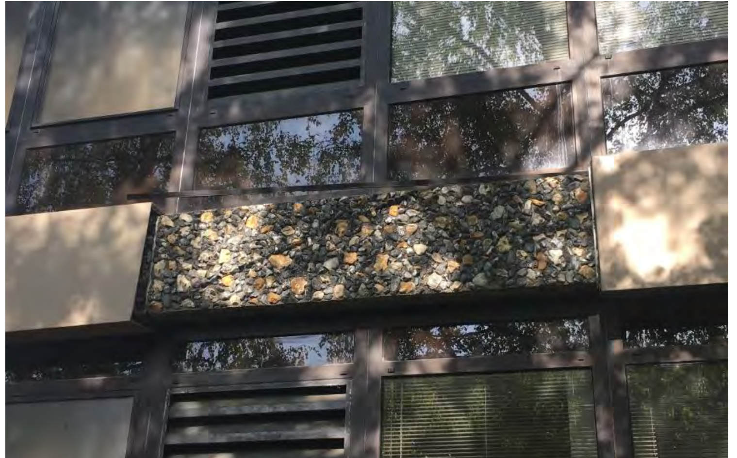
Overcladding removed to show original precast concrete cladding
