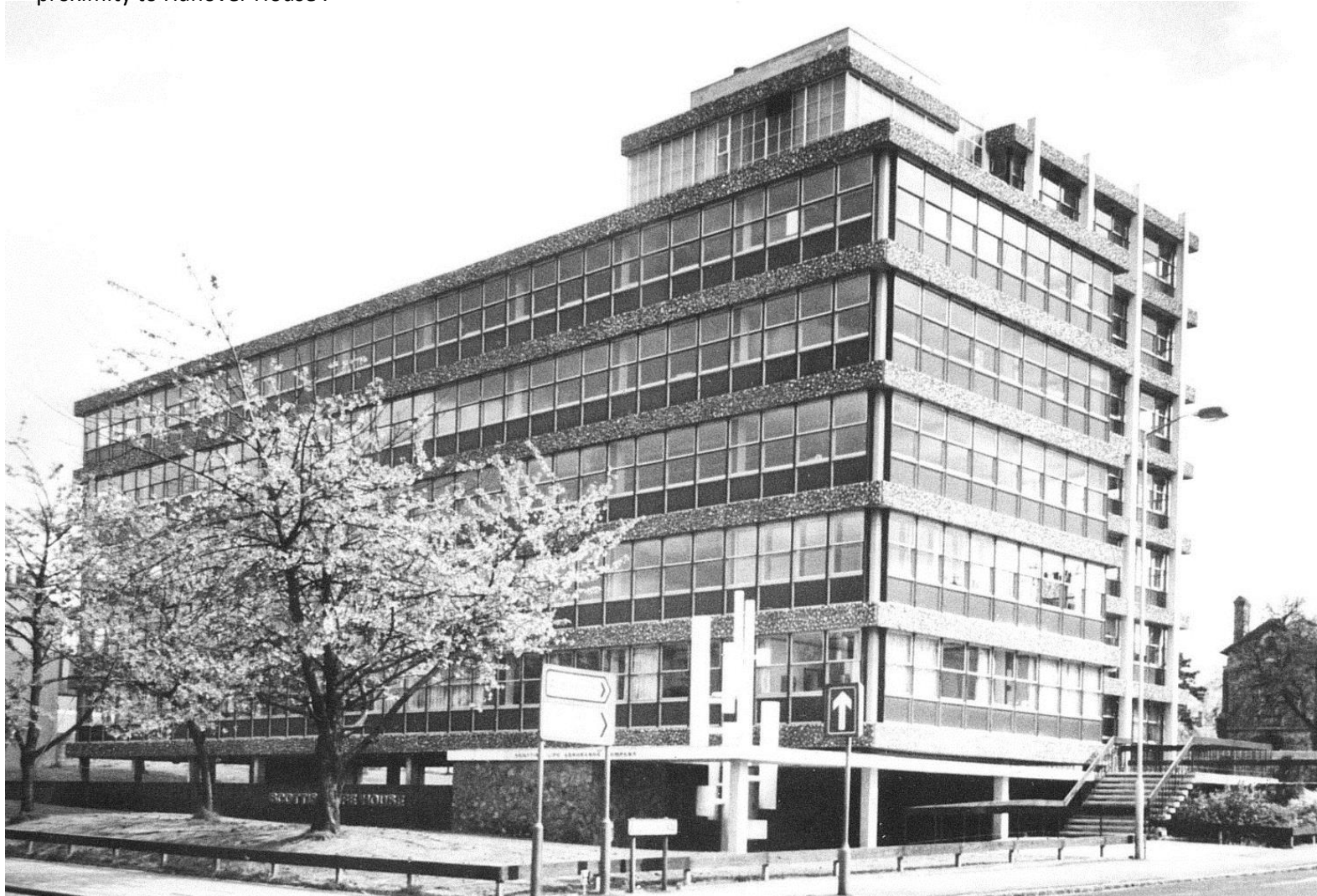
Archive image with the original precast facade.
