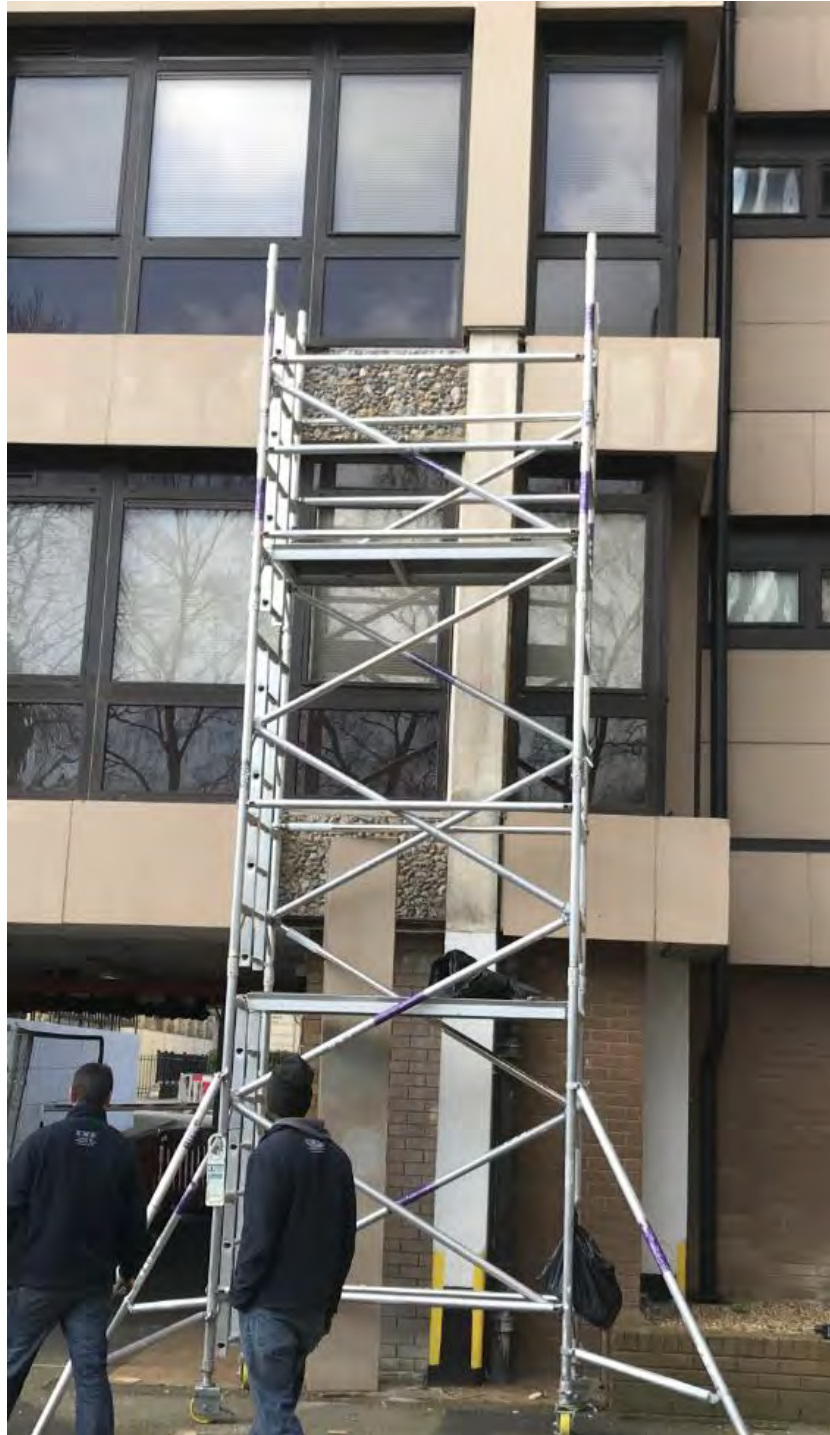
Overcladding removed to show original smooth concrete columns
