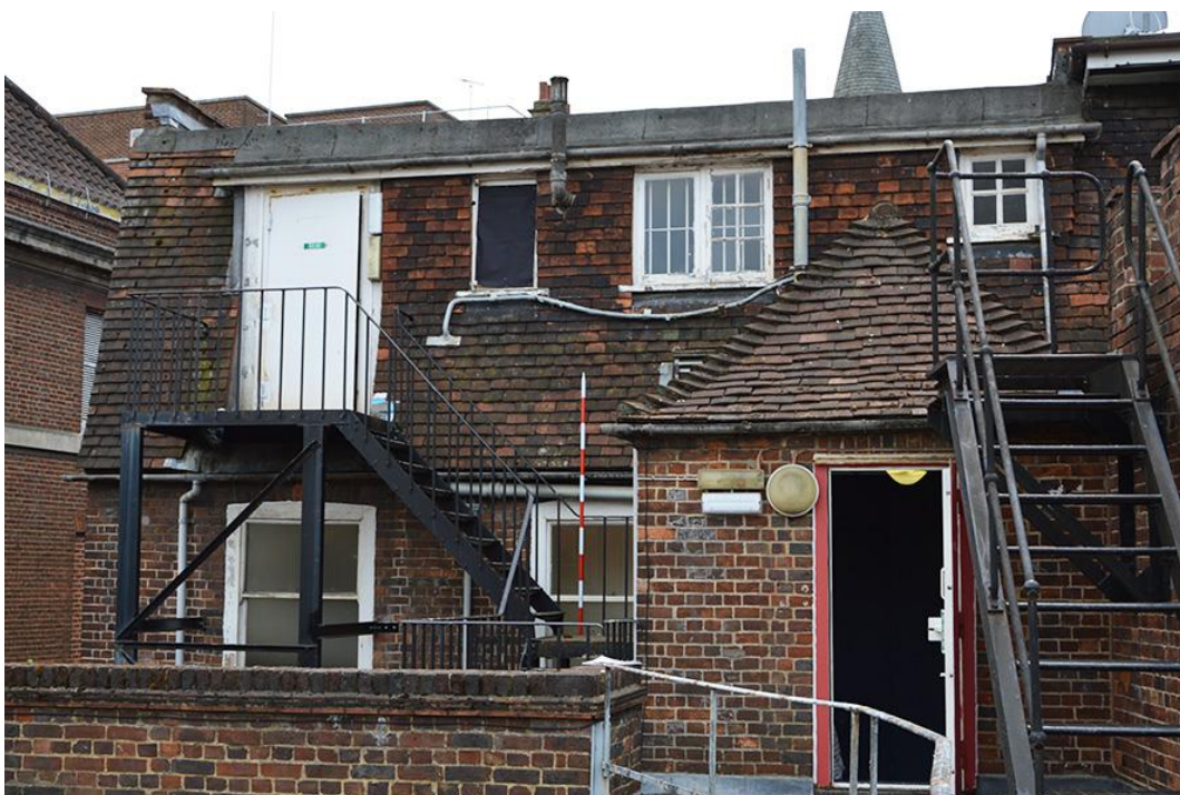
Plate 8: Northern elevation of main building from north
