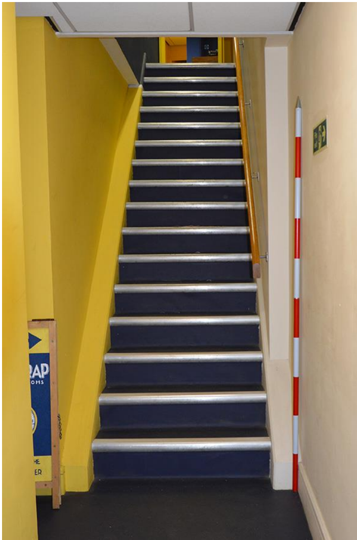
Plate 10: Ground to first floor staircase in rear section of building
