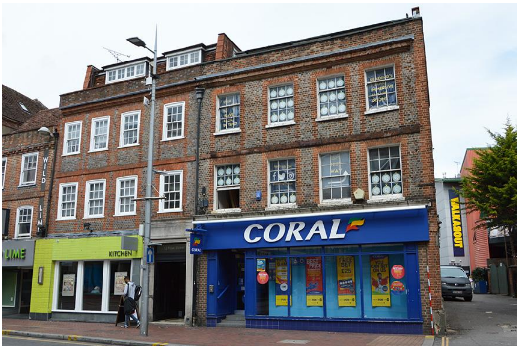
Plate 1: Friar Street elevation of 11 (right) and 12 (left) Friar Street from the south east
