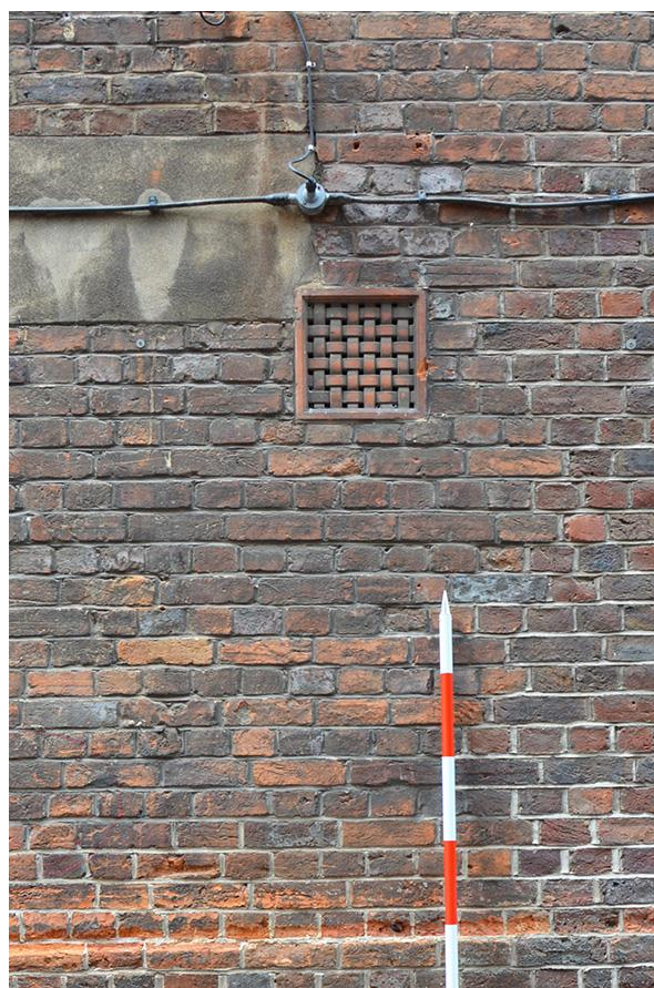
Plate 4: Wiston Terrace elevation, woven terracotta ventilation grill
