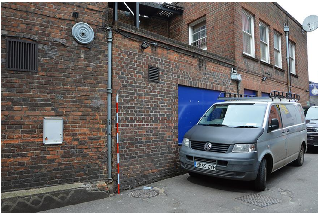
Plate 9: Wall on Wiston Terrace proposed to be demolished
