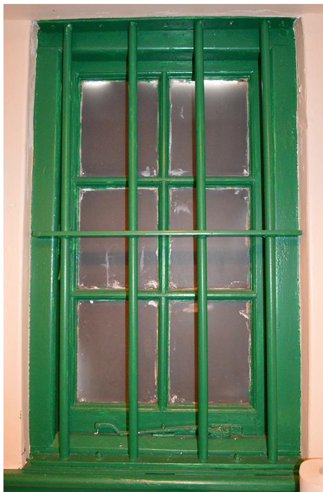
Plate 13: Original bathroom casement window on third floor
