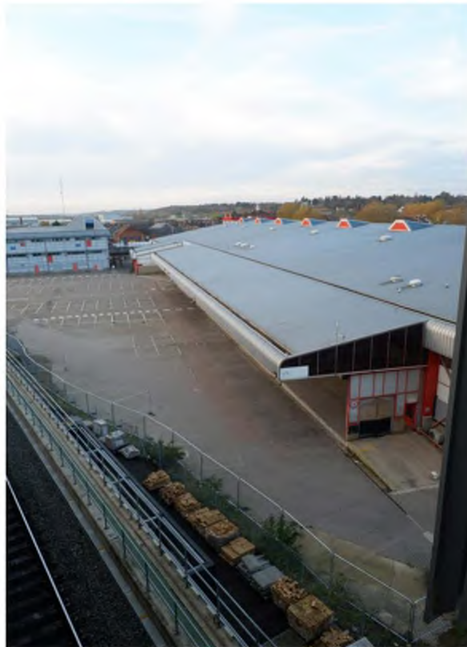
Elevated view from Reading Station
