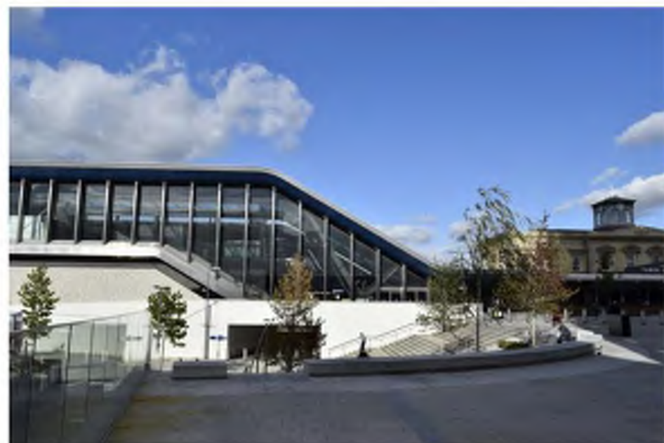
Southern entrance to pedestrian tunnel
