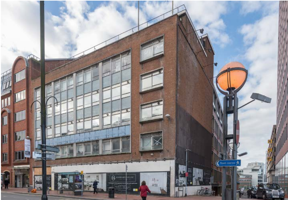
Existing vacant building
