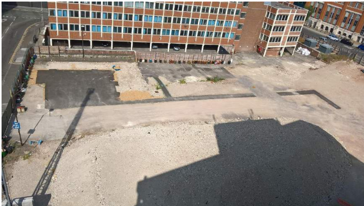
Plate 2 – Compound area located between Garrard Street and Station Hill with crushed aggregate stockpiles where Western Tower was previously demolished.
