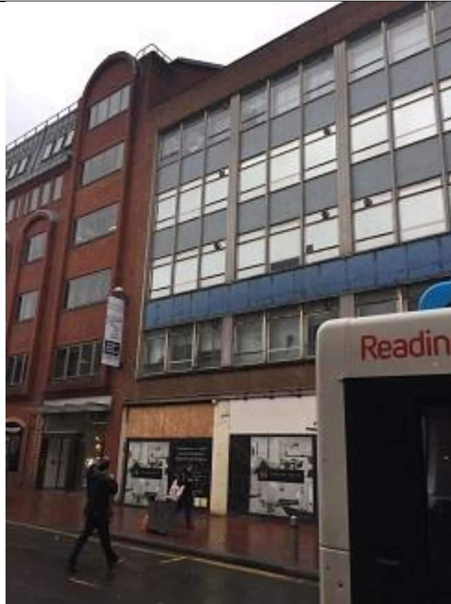
Figure 4: Adjoining property to the south, 27 Station Road.
