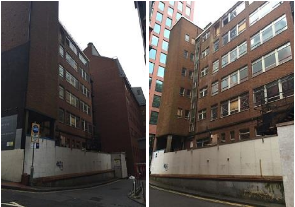
Figure 3: Rear elevation of the property.
