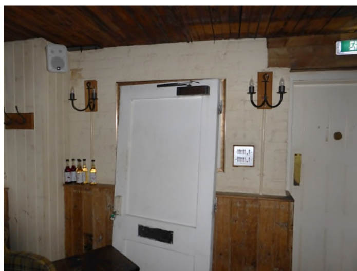
Figure 26: Possible infilled door opening to the room on the south-west side of the ground floor
