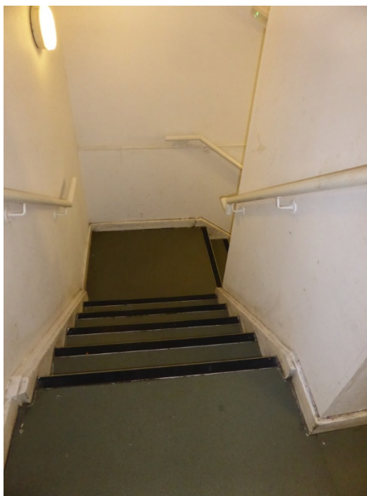
Figure 22: Modern staircase at the western end of the first floor
