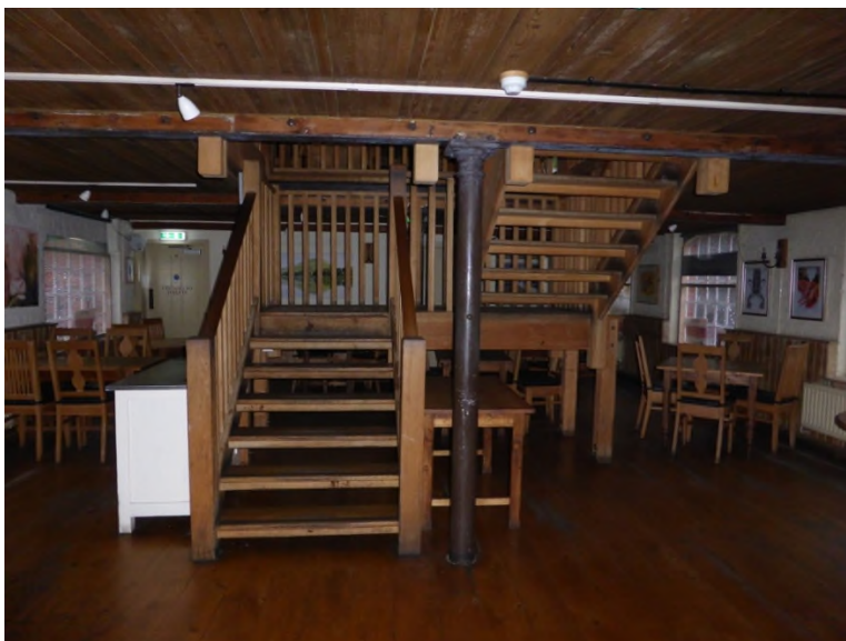
Figure 28: Cast iron column and steel beam and modern staircase on the ground floor
