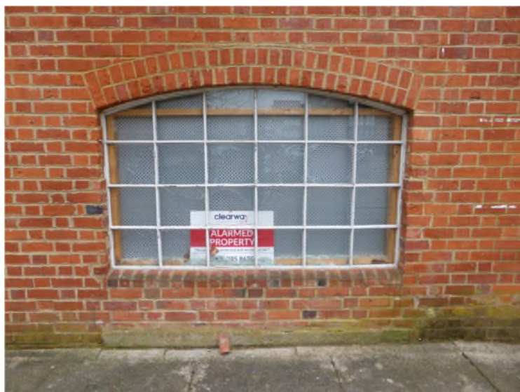
Figure 17: Replacement window at the eastern end of the ground floor
