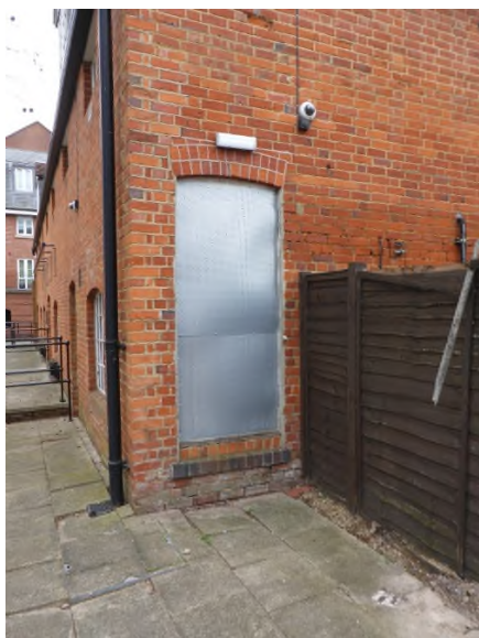
Figure 15: Original door opening on the west elevation
