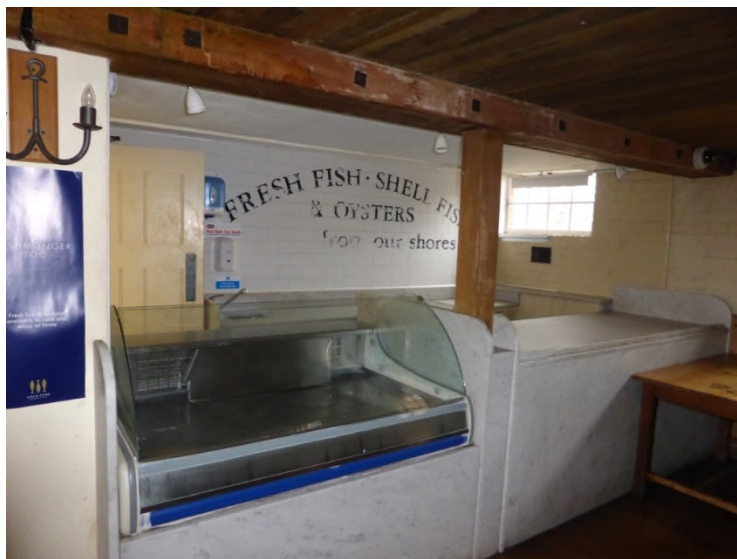
Figure 21: Boxed in beam on the first floor
