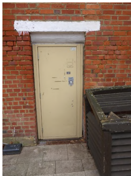
Figure 16: 20 th century door opening on the west elevation
