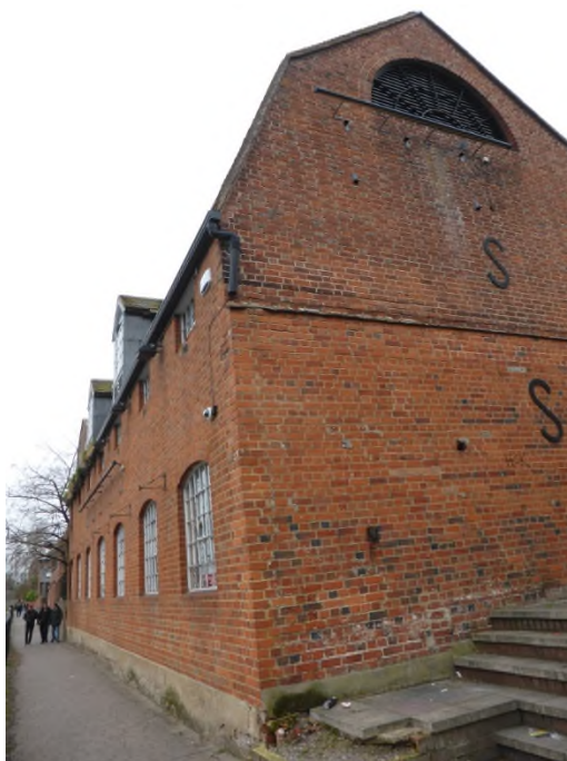
Figure 12: Oblique view of the south and east elevations
