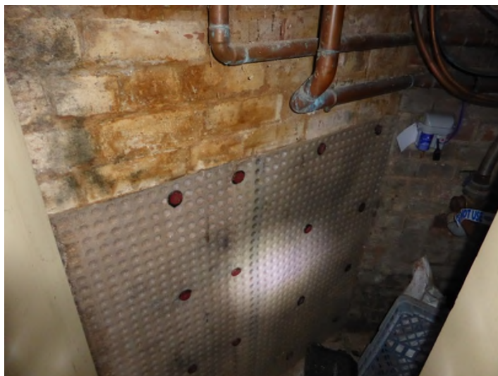
Figure 25: Corner chimney breast in the room on the north-west side of the ground floor
