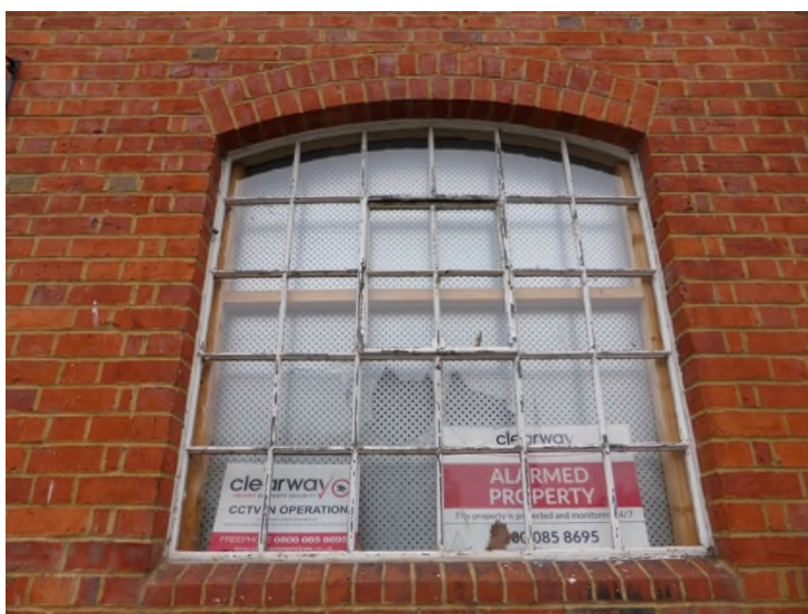
Figure 13: Typical galvanised steel window on the south elevation
