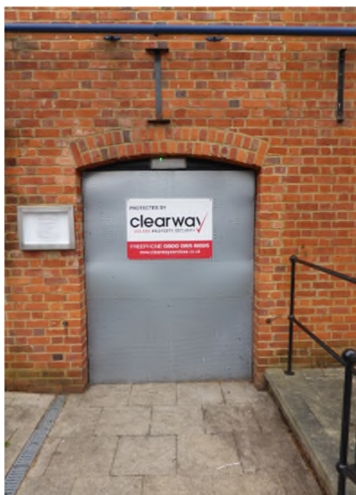
Figure 18: Post-1990 door opening in the position of former external steps to the first floor
