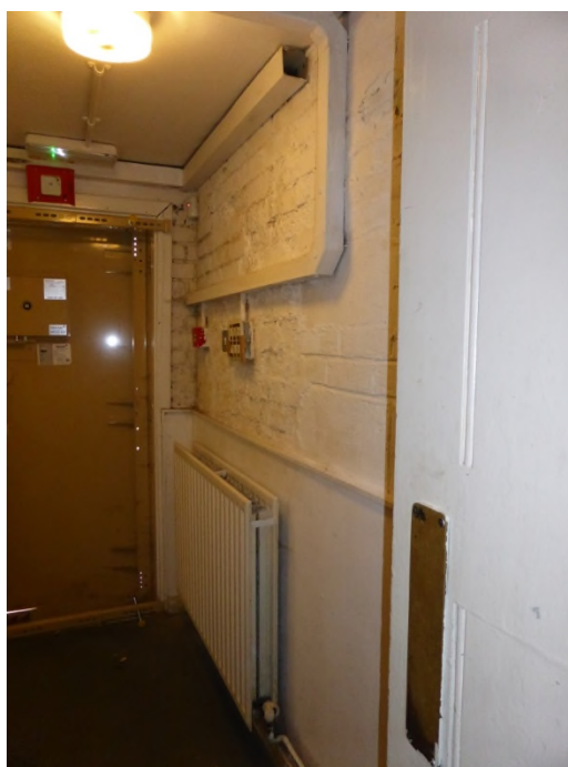
Figure 24: Brick partition to the two rooms at the western end of the ground floor
