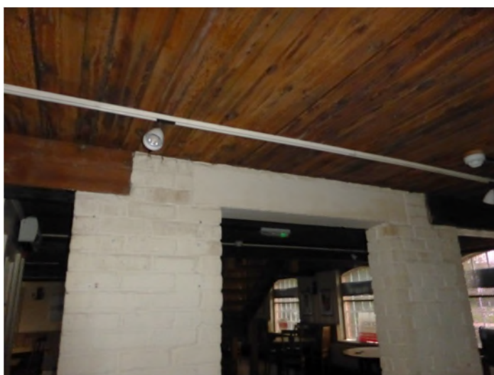
Figure 27: Altered brick partition towards the centre of the ground floor
