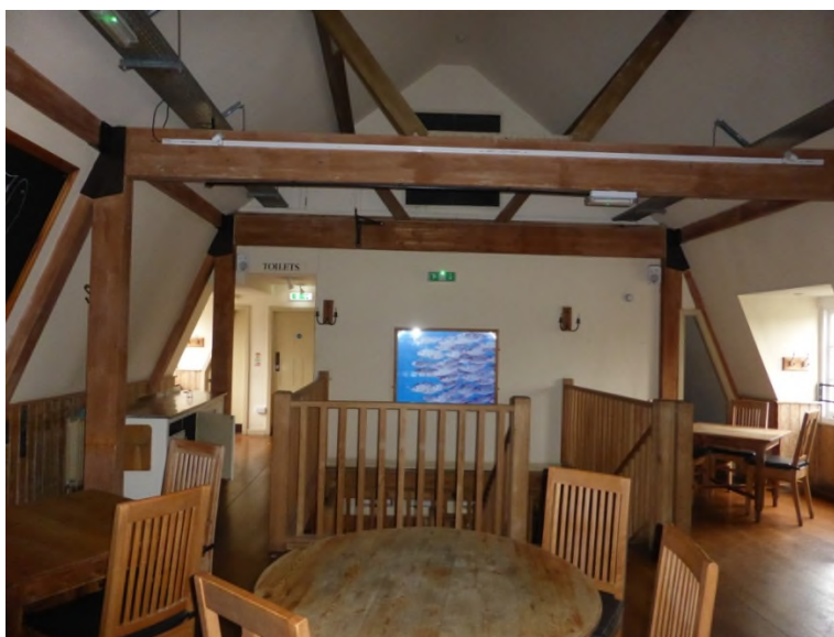
Figure 20: Replacement roof structure on the second floor
