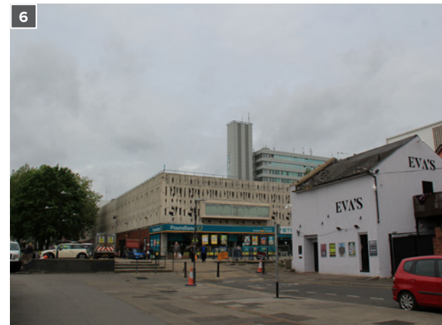
View looking West towards the existing centre with the vacant Eva's nightclub on the right
