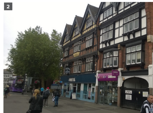
Existing buildings on St Mary's Butts
