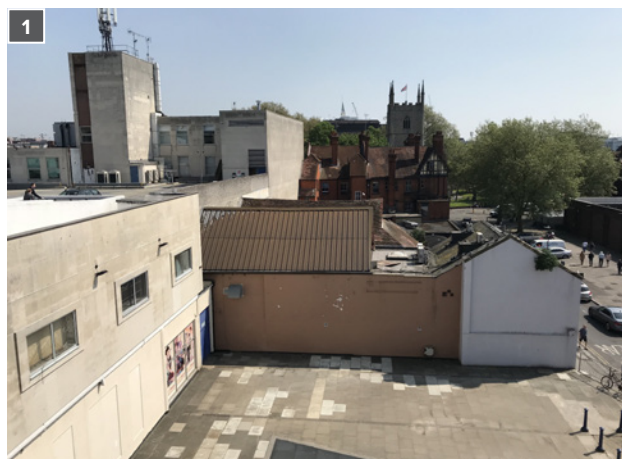
Rooftop view looking East across the existing buildings to be demolished towards Reading Minster
