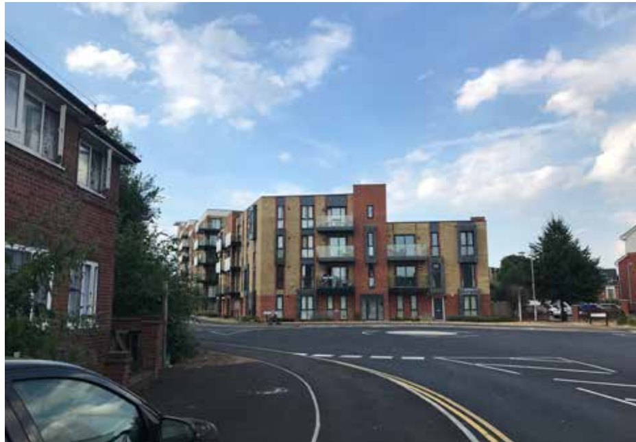
Figure 6.4 Recent development in Character Area A (Bellway scheme).
