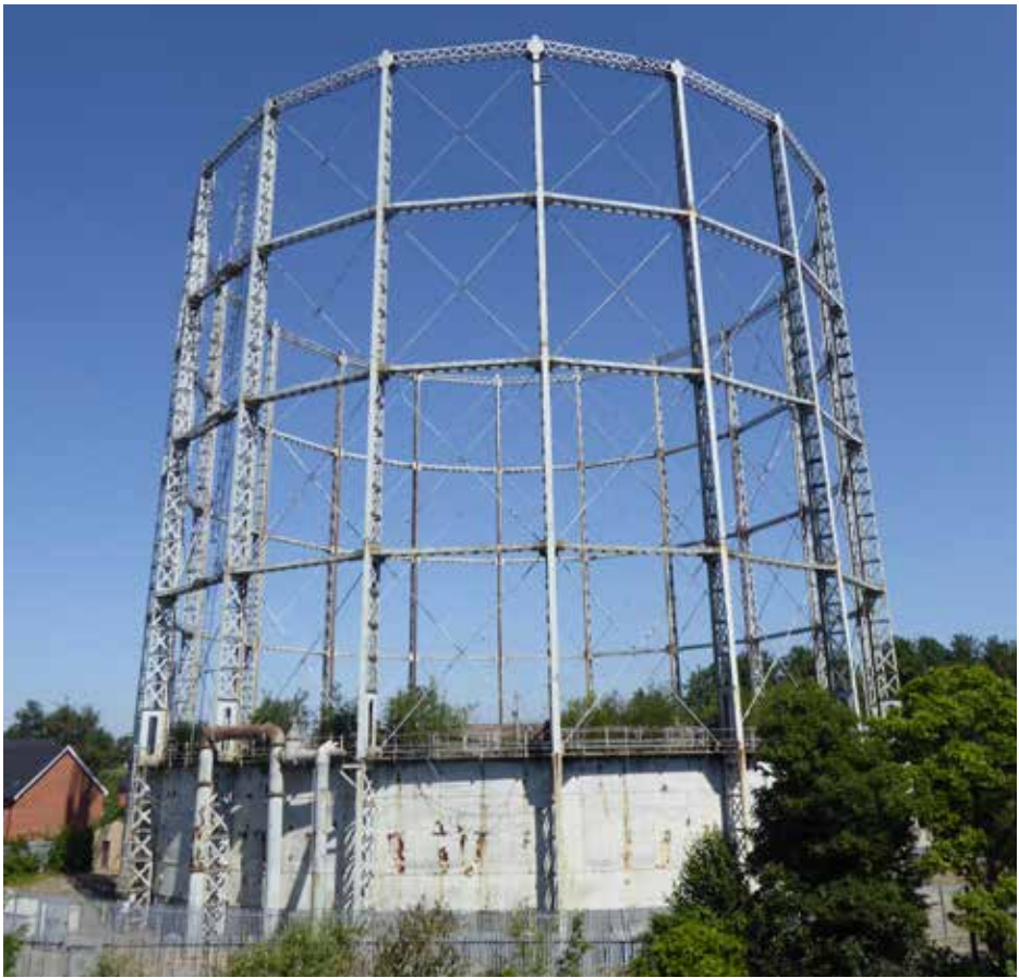
Figure 5.2 GH4 at the east end of Alexander Turner Close, 2018.
