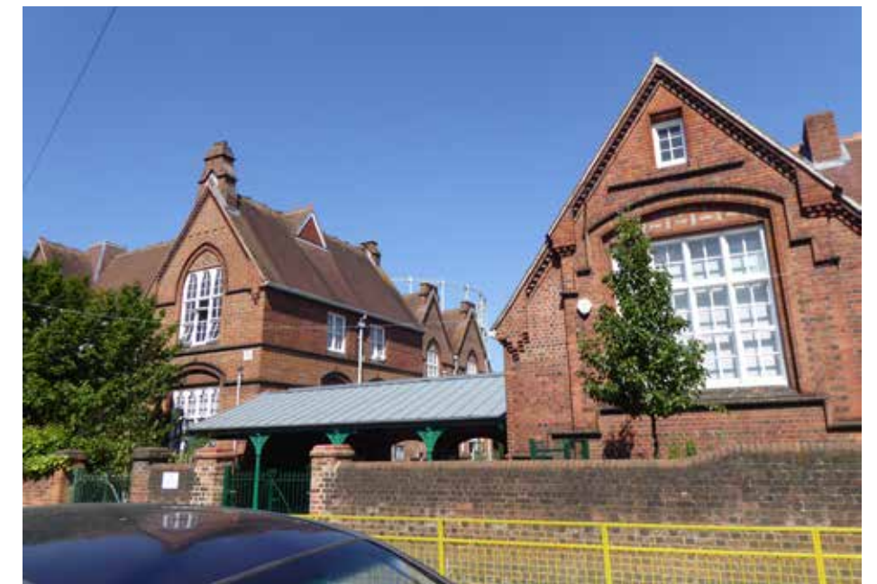
Figure 5.4 The south elevation of the first school building at Newton School (Grade II)
