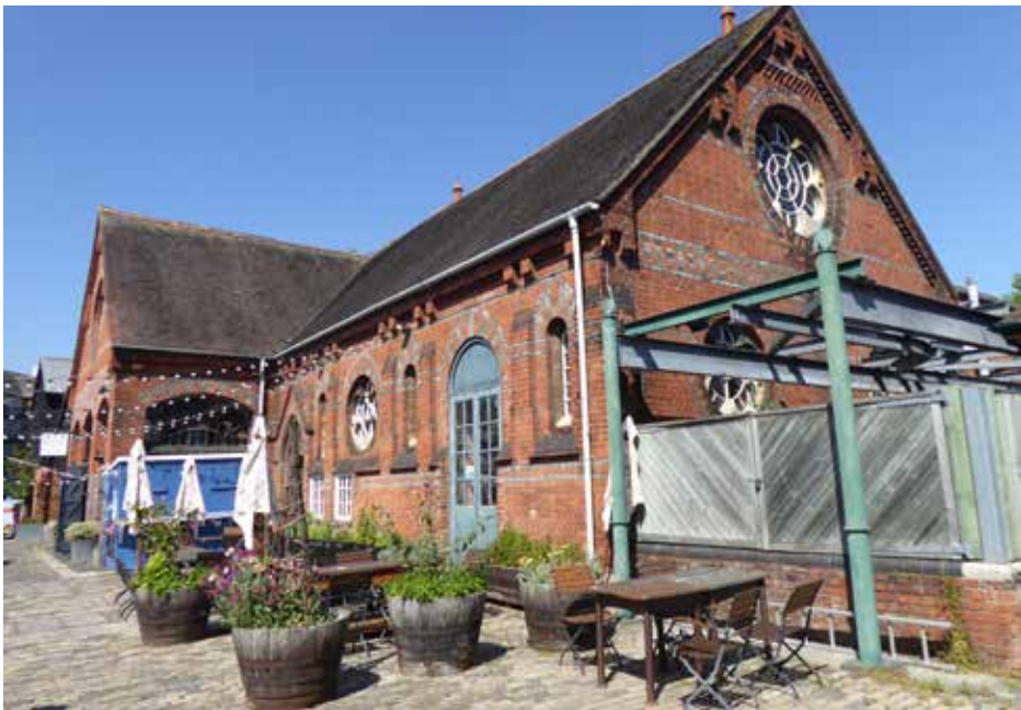
Figure 5.10 The south and east elevation of the Engine House (Grade II).
