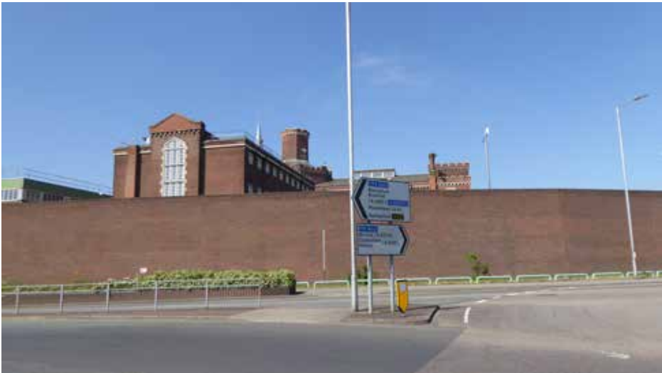
Figure 5.15 Reading Gaol (Grade II) from the north east.
