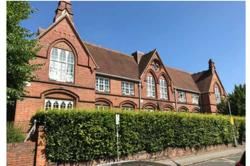
Figure 5.3 The south elevation of the first school building at Newton School (Grade II).
