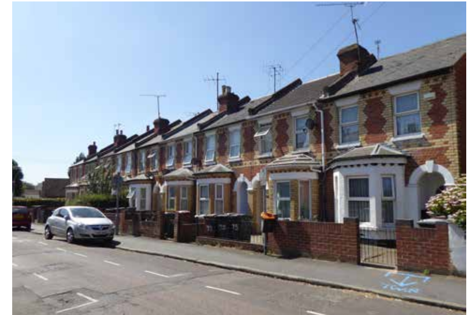
Figure 6.7 Late 19th century character of residential development in Character Area B.
