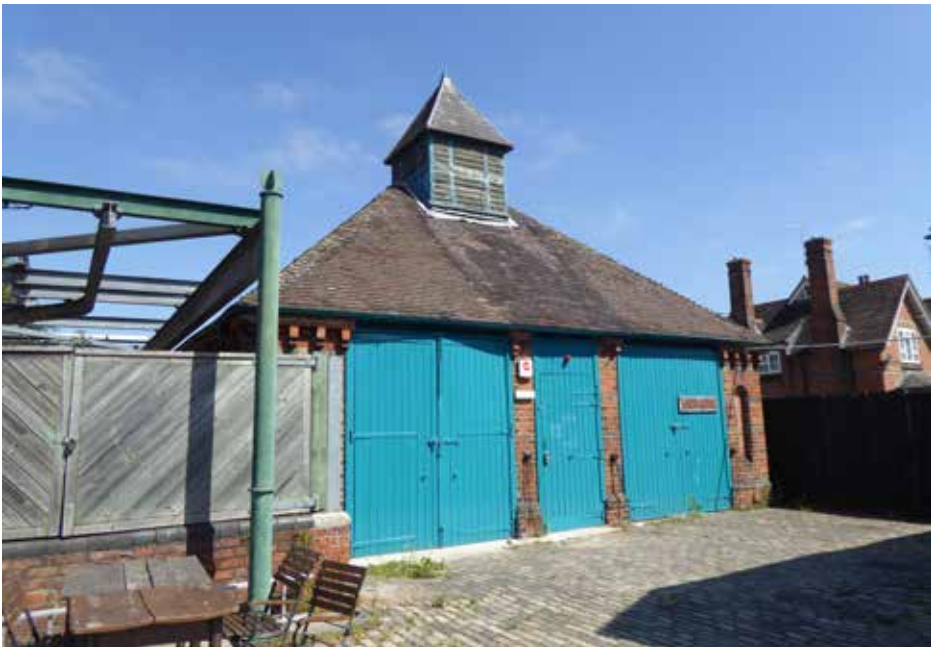
Figure 5.9 The south elevation of the Screens House (Grade II).
