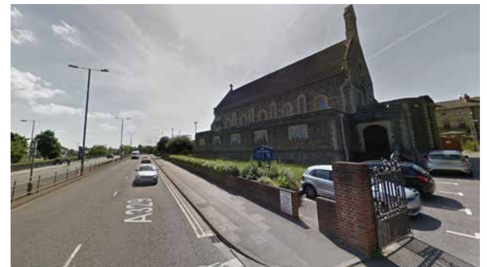
Figure 5.14 The view looking towards the Site from Forbury Road with the Church of St James to the right.
