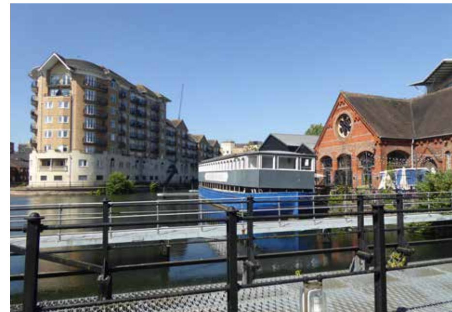
Figure 6.11 Typical mid-late 20th century development in Character Area C.
