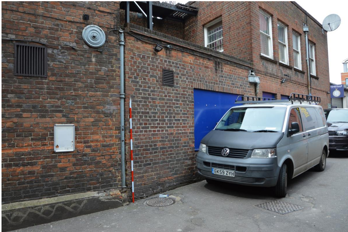
View from Wiston Terrace looking towards Friar Street photo: Shona Robson Glyde - Elmwood Heritage
