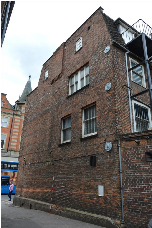
Corner of building looking from Wiston Terrace towards Friar Street
