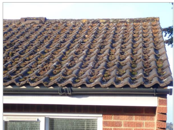
Photo 12 Roof tiles, front elevation
