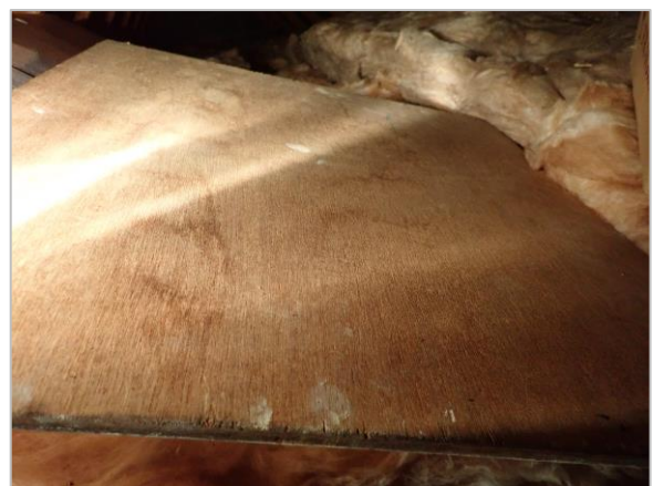
Photo 6 Boarding in loft
