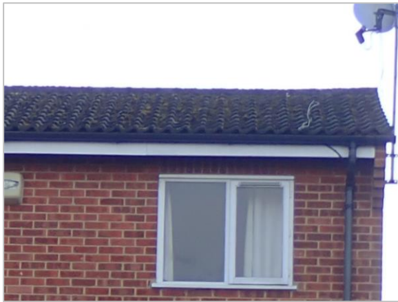
Photo 13 Tiles to rear elevation
