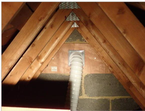
Photo 9 Vent pipe to eastern gable end
