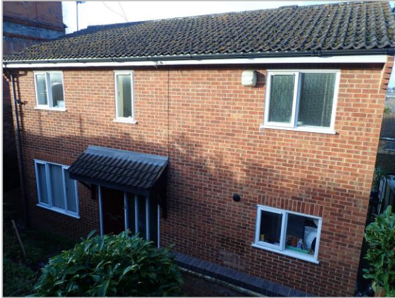
Photo 1 Front (south) elevation
