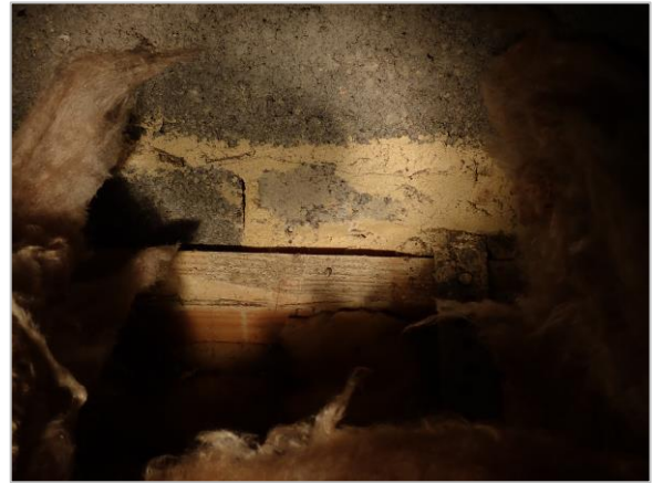
Photo 8 Floor beneath gable apex
