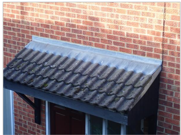
Photo 16 Porch roof in good condition; no gaps to flashing
