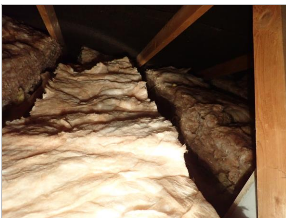
Photo 5 Insulation in loft
