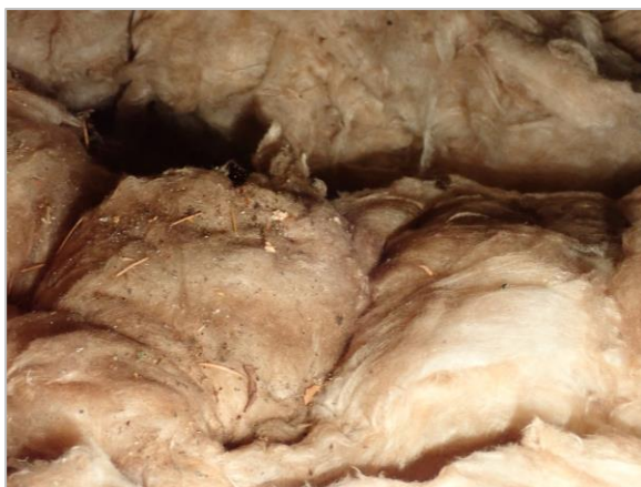
Photo 11 Insulation beneath ridge vent
