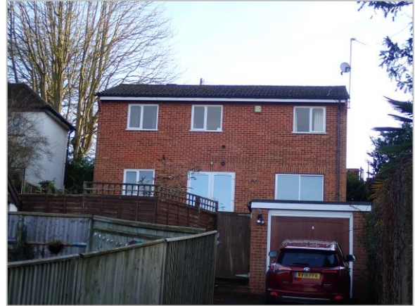
Photo 2 Rear (north) elevation
