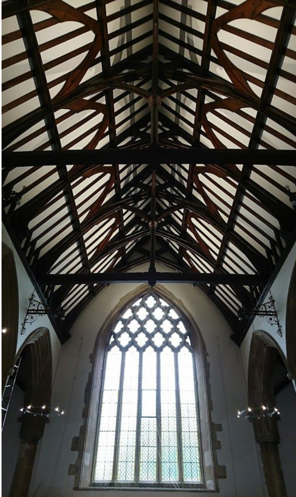
Above: nave roof and west window; note elaborate wrought iron light brackets.
