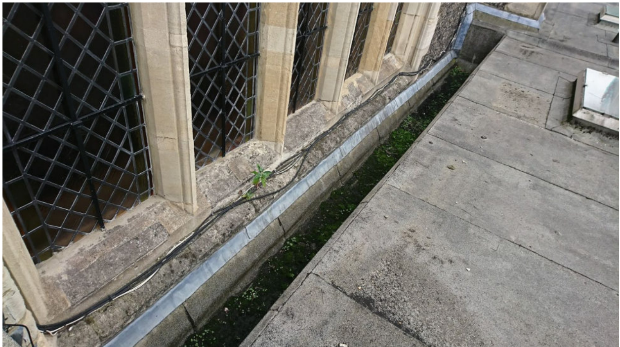
Below: junction of 1972 roof with renewed 14th century west window
