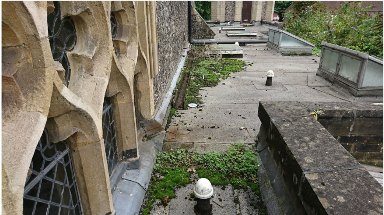
Above: flat roof to 1972 north link and west end extension
