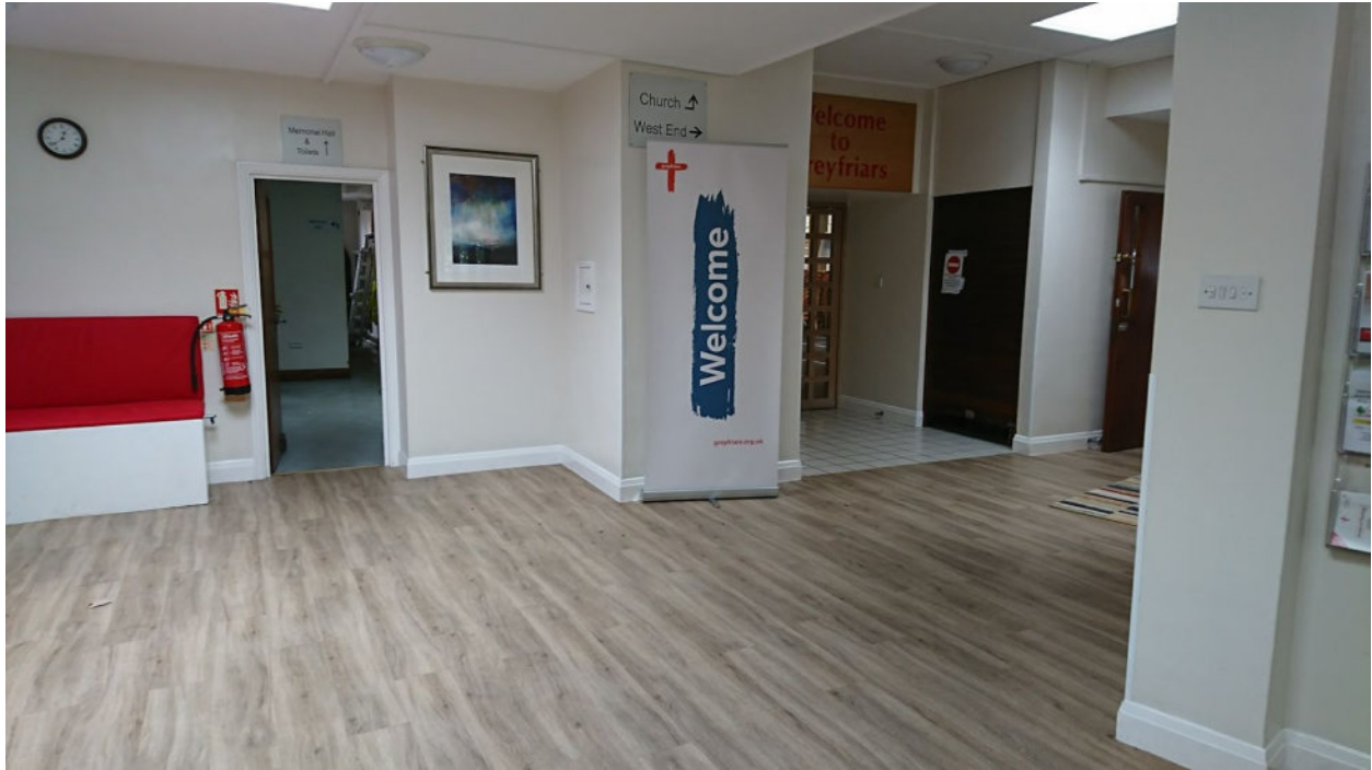
Above: refurbished entrance/welcome area
