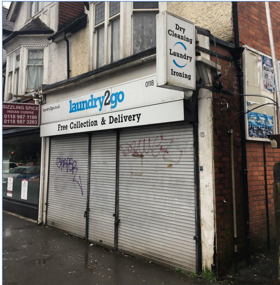
Existing shopfront to be replaced
