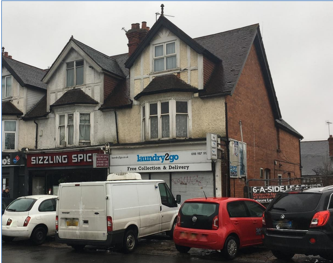
North and west elevations of 60 Christchurch Road, Reading
