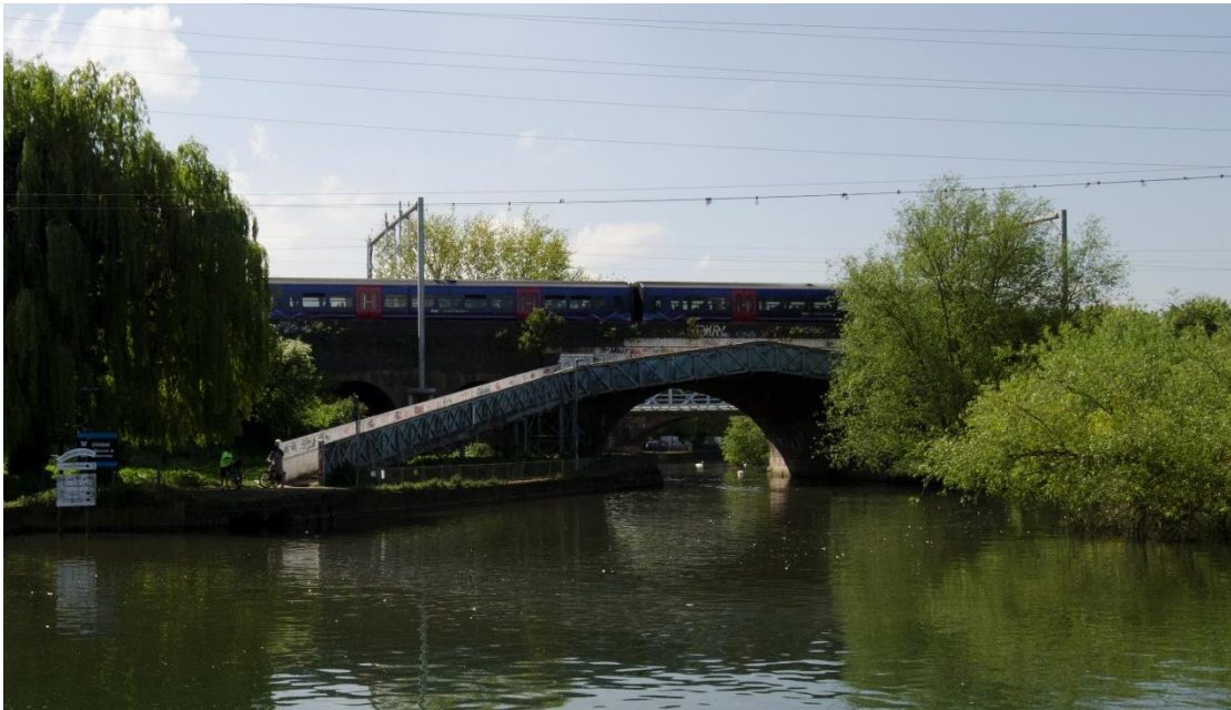
Figure 3.5: Stepped Horseshoe Bridge
