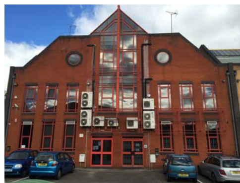
Fig 2: View of site from the rear. (No 10 on left, No 9 on right)
