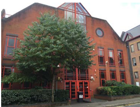
Fig 1: Site from South St (No 9 on left, No 10 on right)
