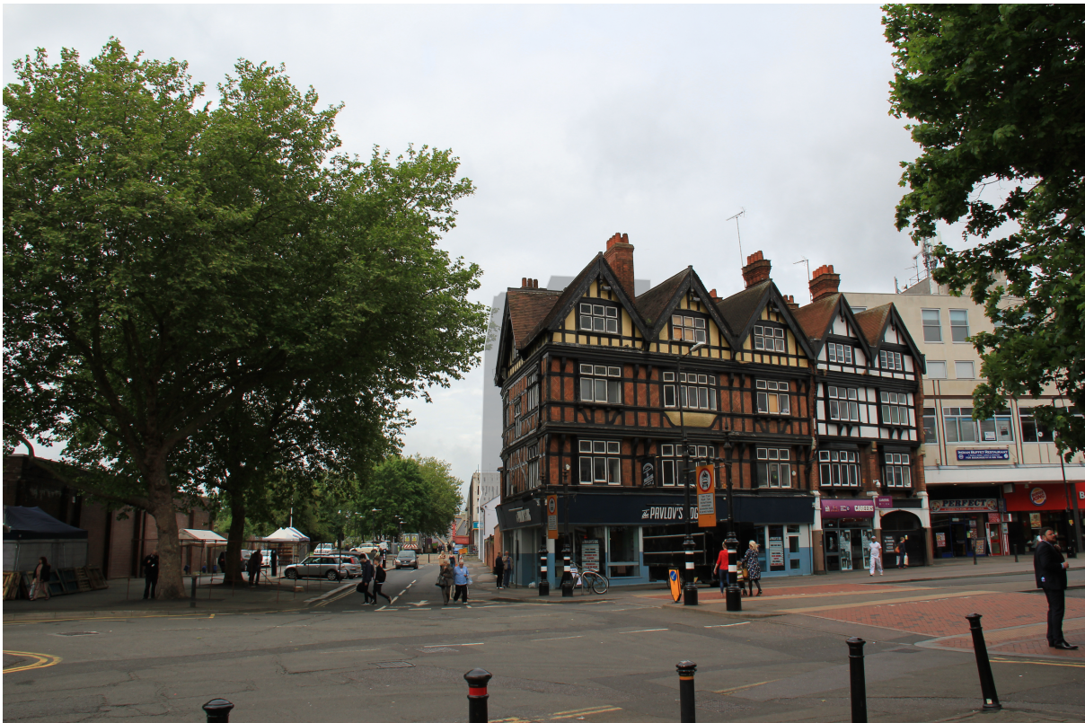
View 1: Looking east towards the site from the church
