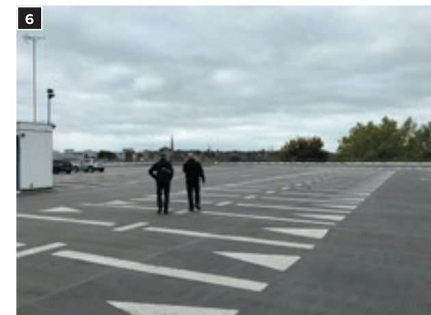
Car Park deck
