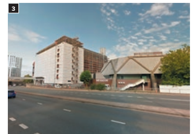
View from the A329 looking towards the Hexagon
