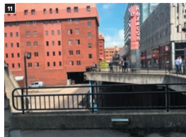
View looking down to the car park access road
