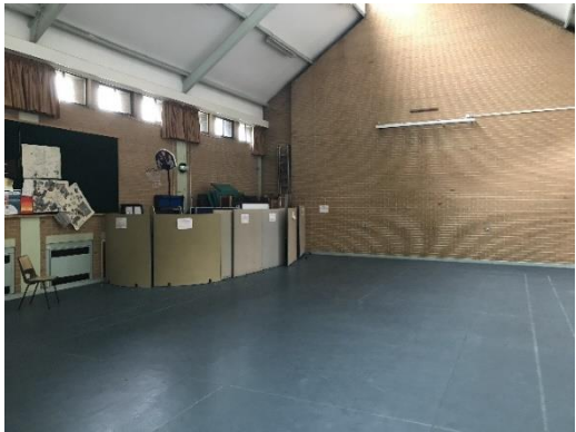
Centre Main Hall
