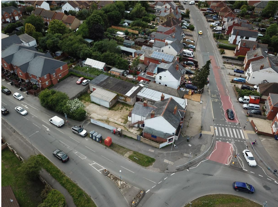
Aerial view of site
