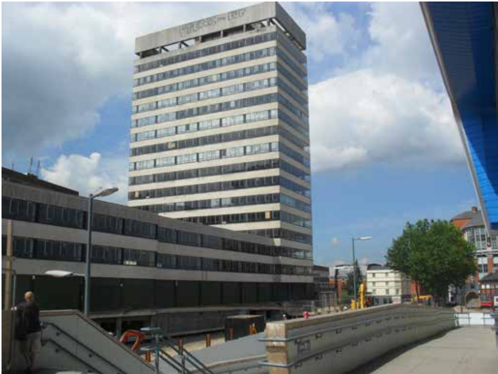
View westwards along Station Hill towards Western Tower and Xafinity House in the northwest corner of the Site.
