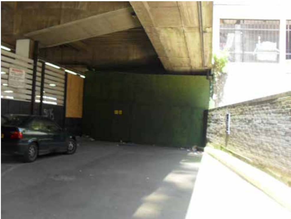
View northwards at the entrance to the underground car park below the Site.
