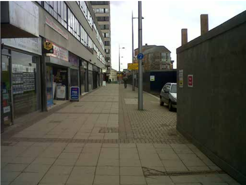
Station Hill Retail Units.
