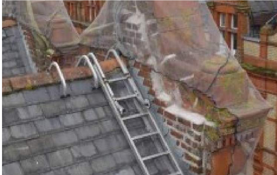
Plate 4.2 Rear of No 12 Gable showing the degree of masonry repair
