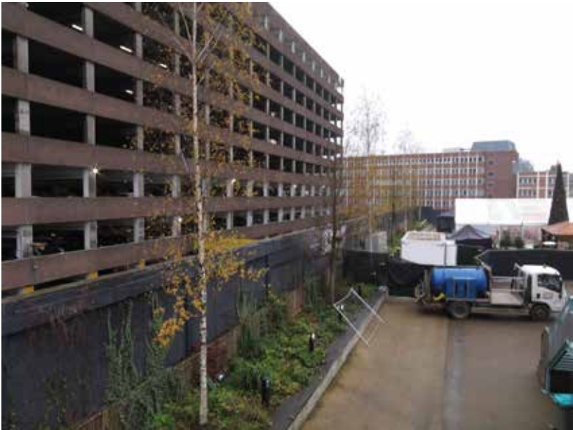
View of Garrard Street Carpark
