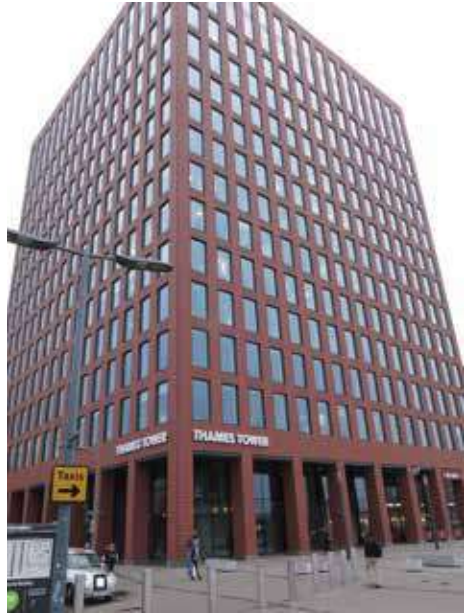
Thames Tower to the east of the Site boundary
