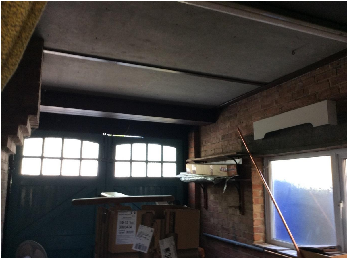
Fig 6. Interior of garage.
