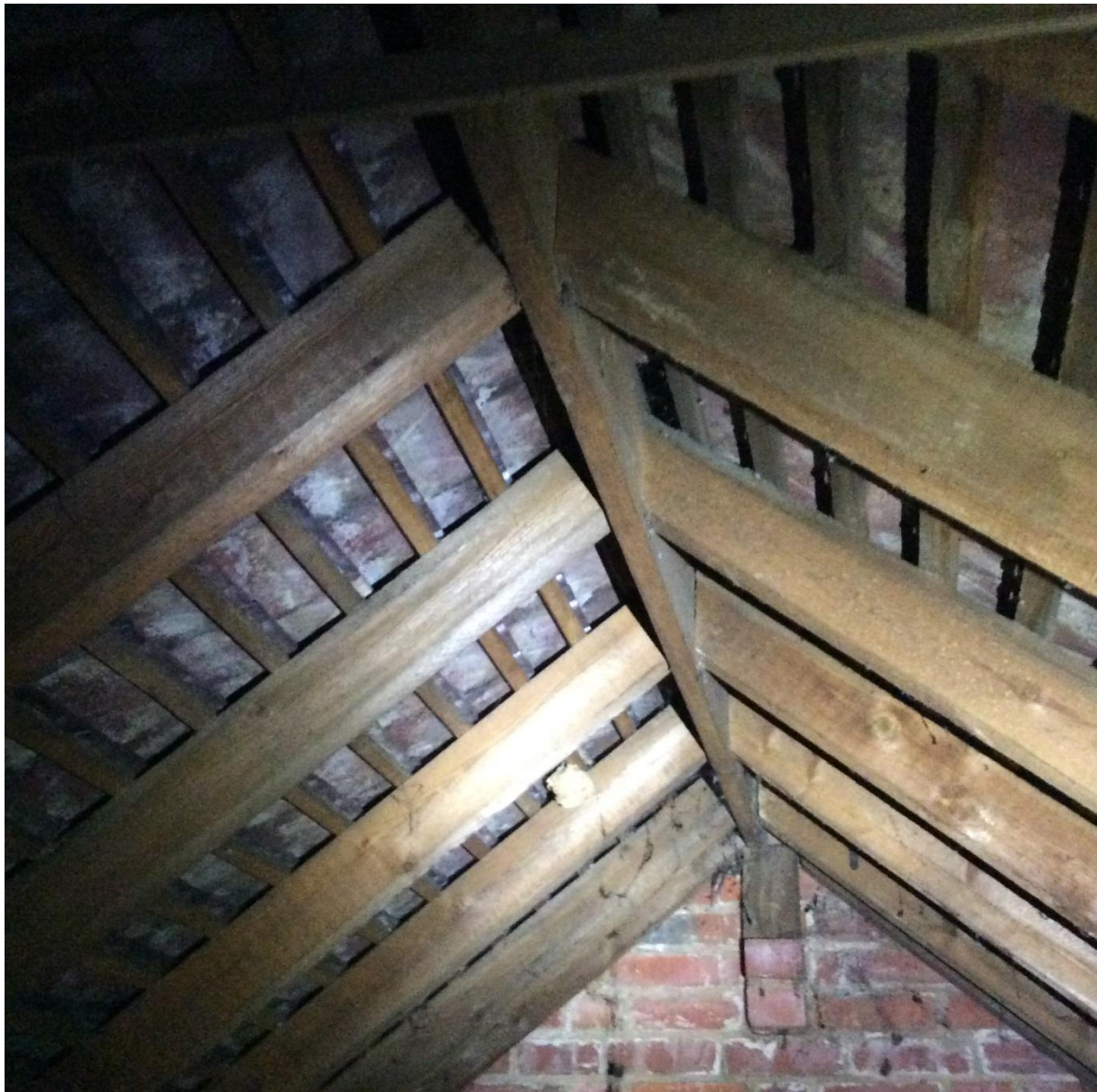
Fig 5. Interior of main loft looking north
