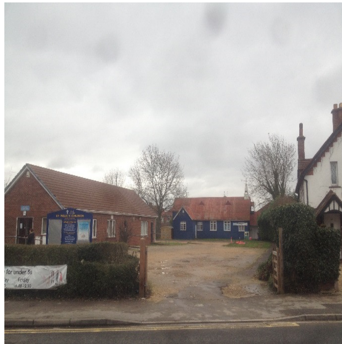
View into the site, Hall on the left and the church distant.
